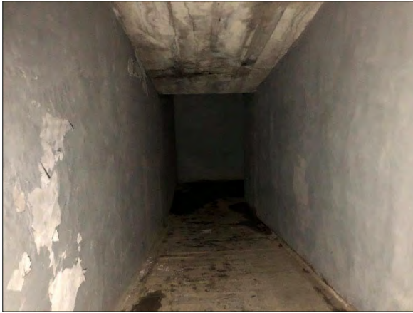
Figures 17 & 18: Failing veneer coverings to ramp walls
