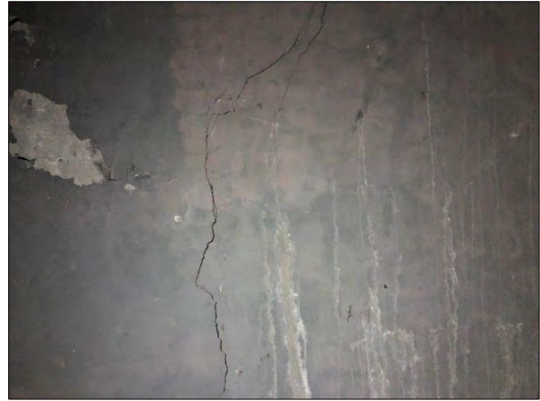
Figures 17 & 18: Failing veneer coverings to ramp walls
