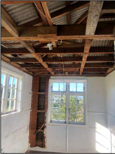
Areas of roof and ceiling framing. Note original timbers and later recycled material.
