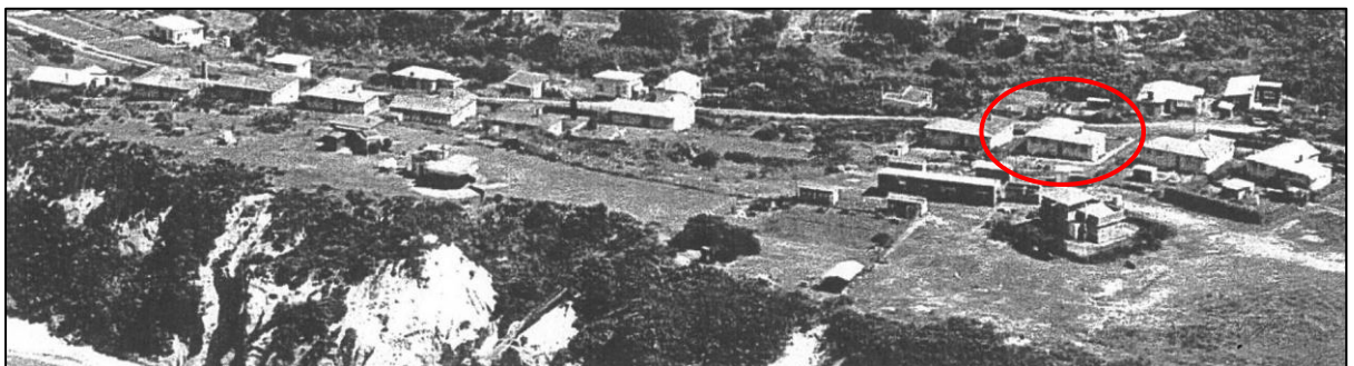
Aerial view showing houses in their relocated position. The house in question is indicated with the red circle with the Battery Observation Post immediately below. The gun emplacements are located centre left. The remaining buildings at the left and right of the photograph have all been demolished.
