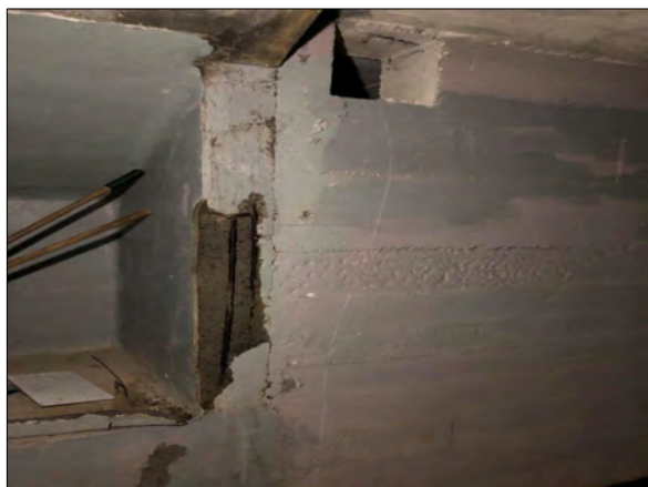
Figures 13 & 14: Damage to Ammunition Niche Corridor walls
