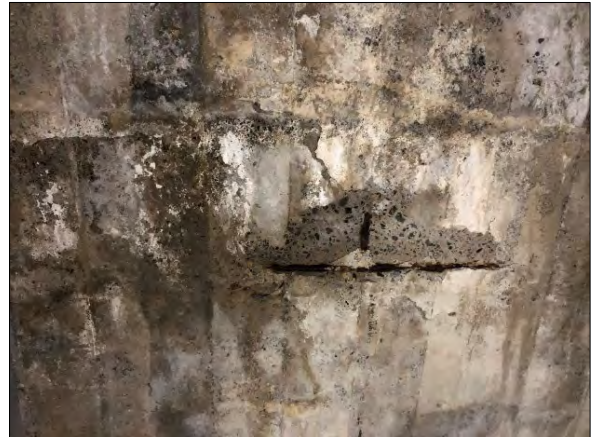
Figures 19 & 20: Water and corrosion staining, concrete spalls to ramp ceilings
