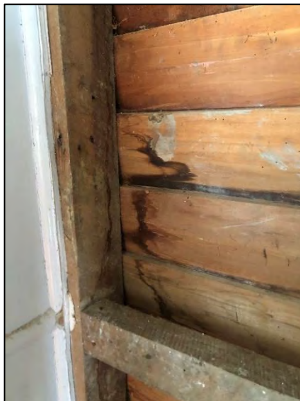
External wall framing. Note water staining on weatherboards.
