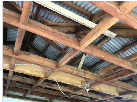
Areas of roof and ceiling framing. Note original timbers and later recycled material.
