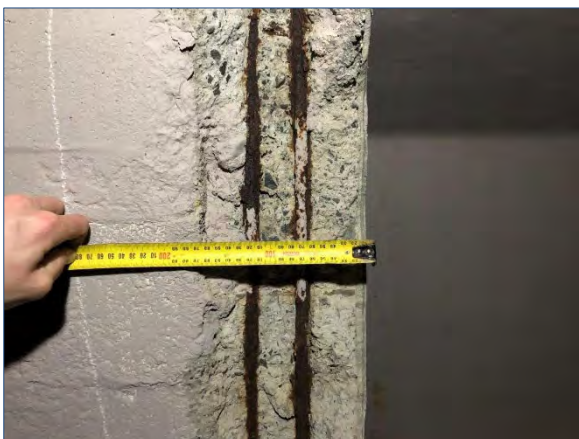
Figures 13 & 14: Damage to Ammunition Niche Corridor walls
