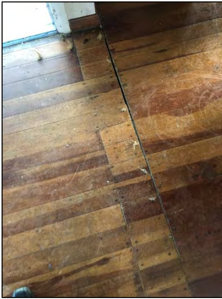
Matai tongue and groove floor boards. Note cut line.
