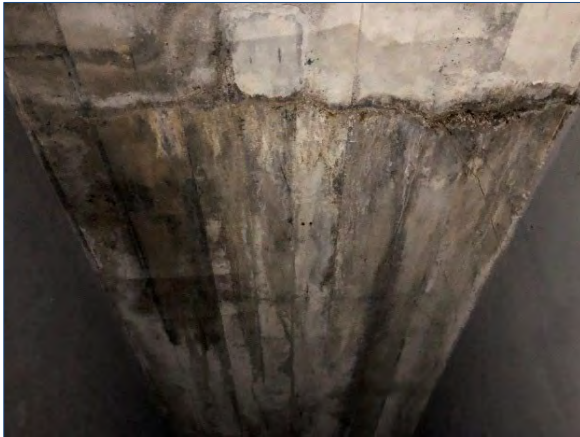
Figures 19 & 20: Water and corrosion staining, concrete spalls to ramp ceilings
