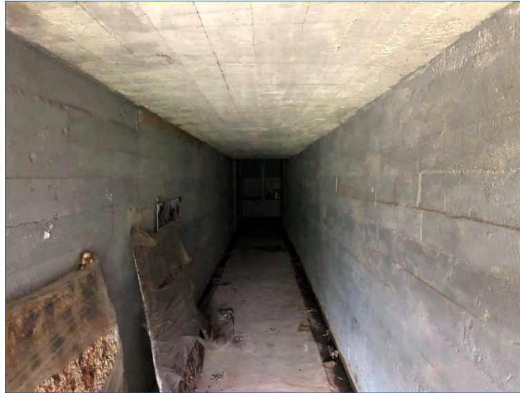
Figure 4: Western Entrance Tunnel
