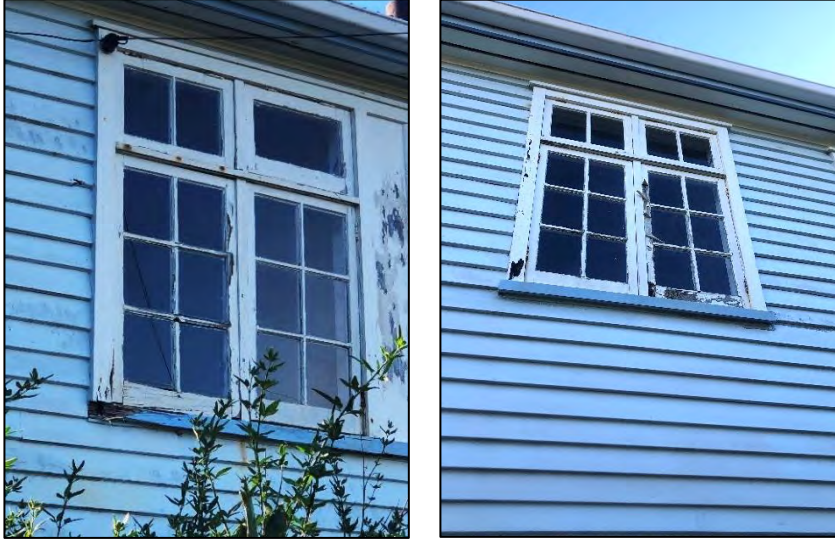
Decay in window joinery, in sill and facing (left) and sash members (right).
