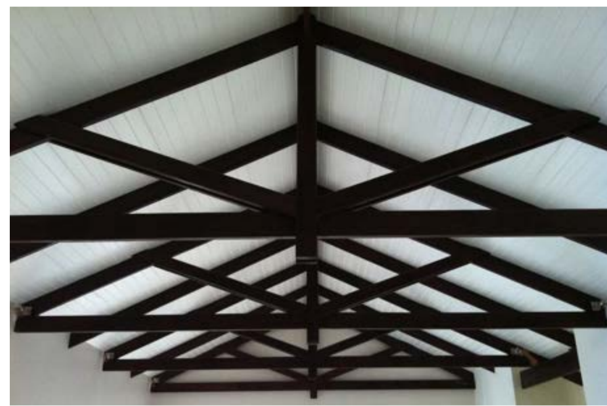
Dark timber trusses
