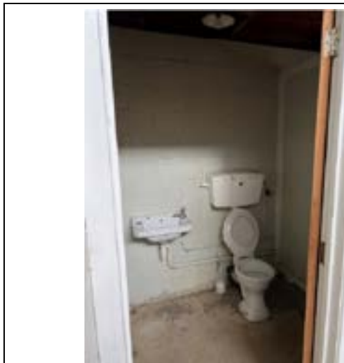
Image 2: Toilets located in the centre of the building are in poor condition. There is no accessible toilet.
