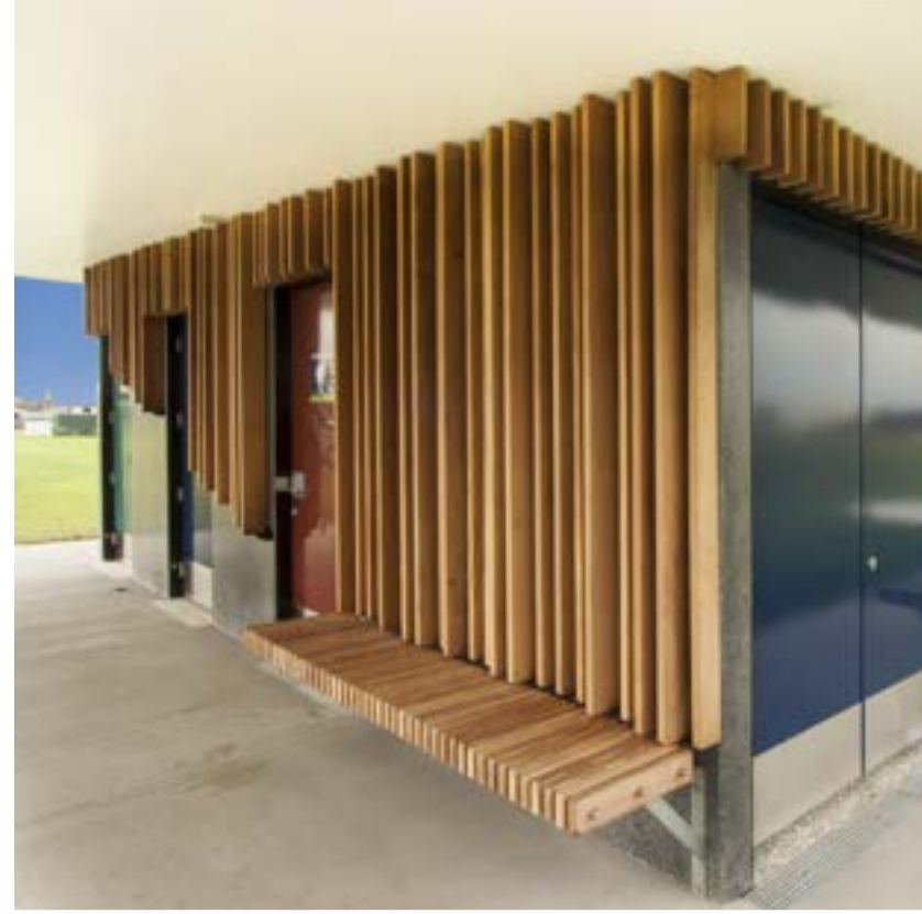
Material palette for north and south facade, using timber battens to create interest
