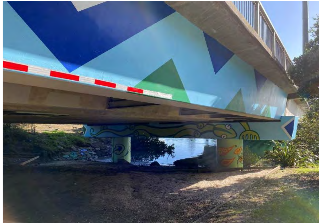
Completed East side with the view beneath
