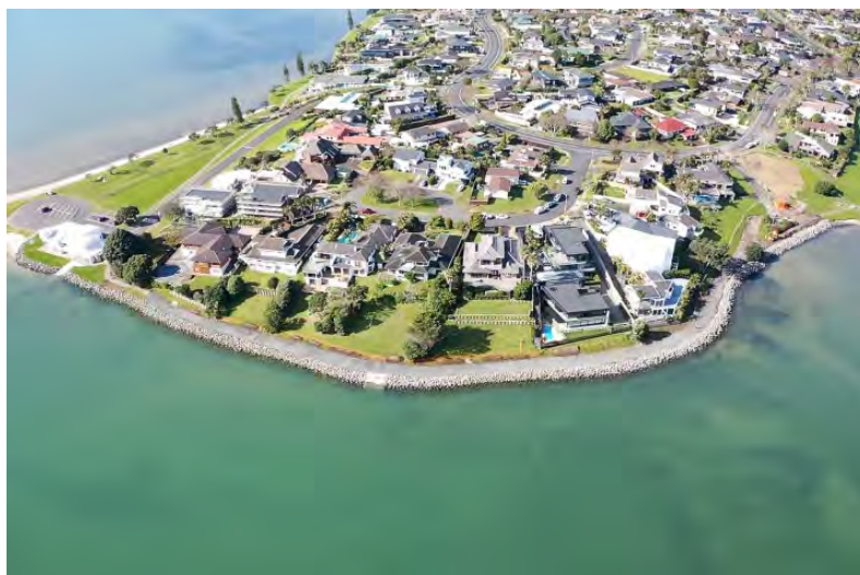
Bramley Drive Seawall
