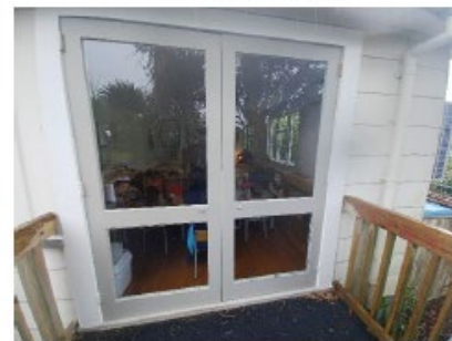
6. Renewed ramp timber barrier.
