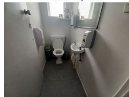
17. Refurbished floor covering in toilet.
