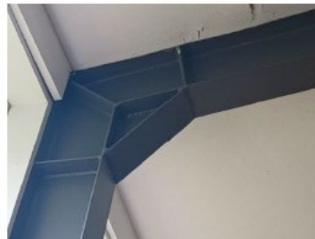
23. Good condition steel portal frame.
