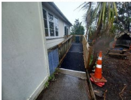
5. Renewed accessible ramp.
