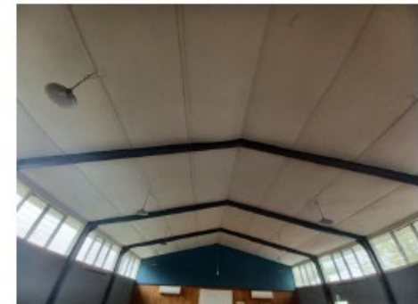
22. Hall ceiling showing steel portal frame.
