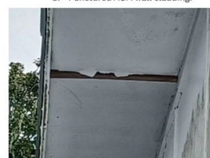
10. Flaking paint soffit lining.
