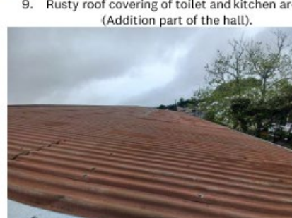
11. Hall area roof covering.
