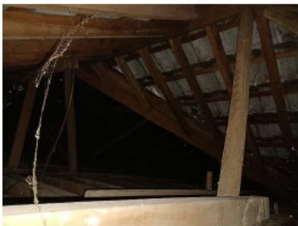
19. Satisfactory timber trusses.
