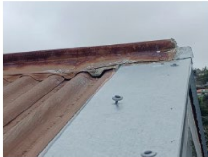
13. Lifting of nails to the barge flashing.
