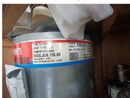
22. Unstrap hot water cylinder.
