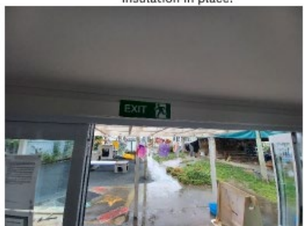
23. Exit sign and recent aluminium bifold door.
