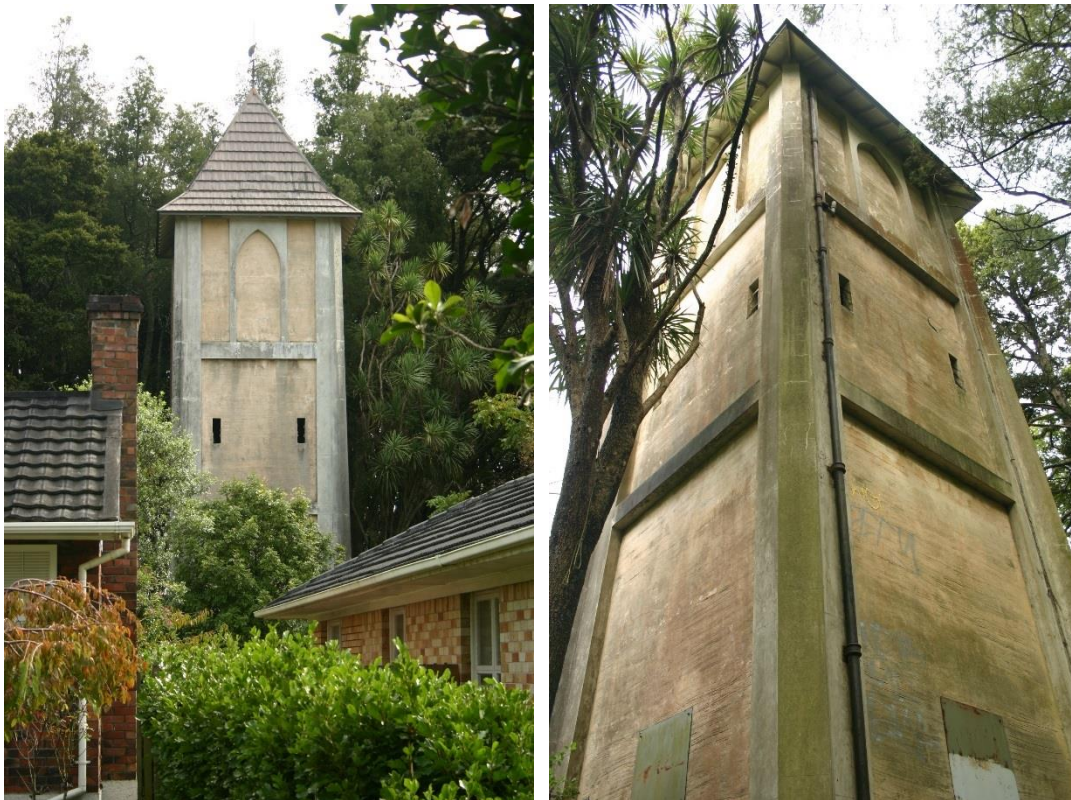
Figure 14: Views towards the water tower. Photos Matthews & Matthews Architects Ltd 2008
