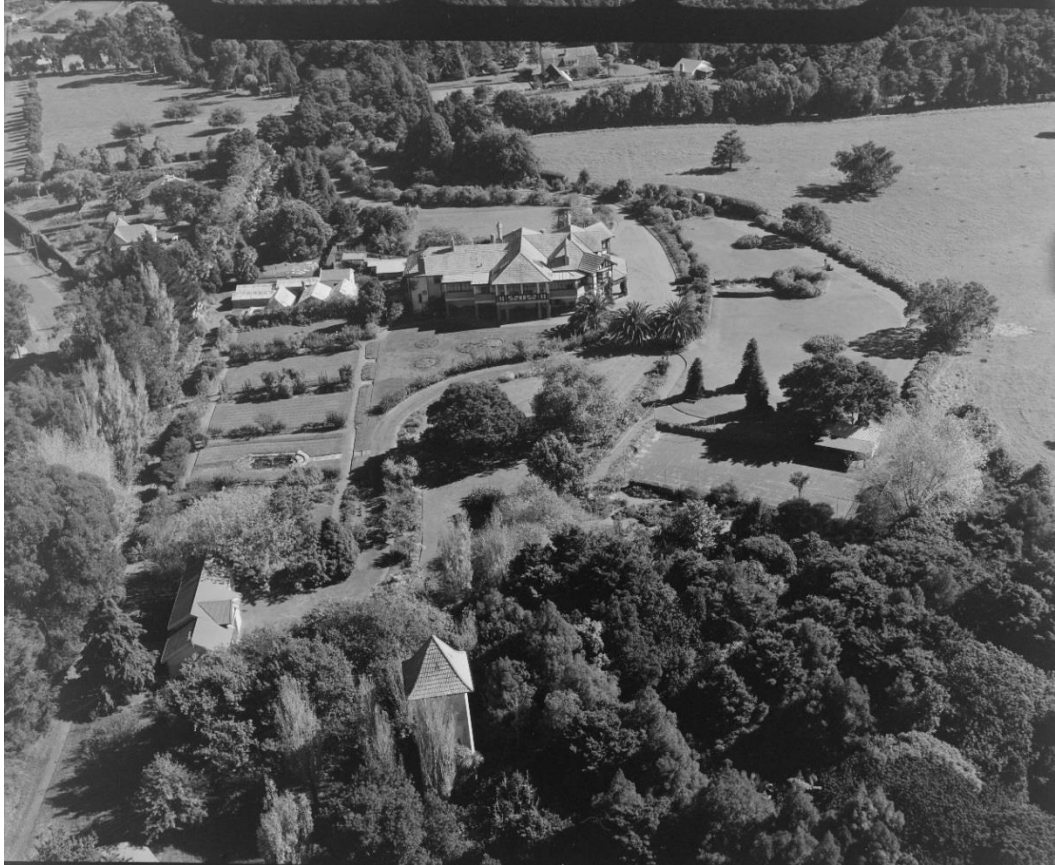
Figure 33: Aerial photograph taken by Whites Aviation showing the Nathan Homestead and garden from the east, April 1949. Nathan home, Manurewa, Auckland. Ref: WA-20228-F. Alexander Turnbull Library, Wellington, New Zealand. /records/23213506.
