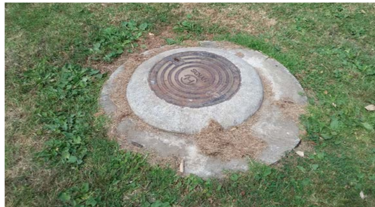
Exposed manhole on grassed area
