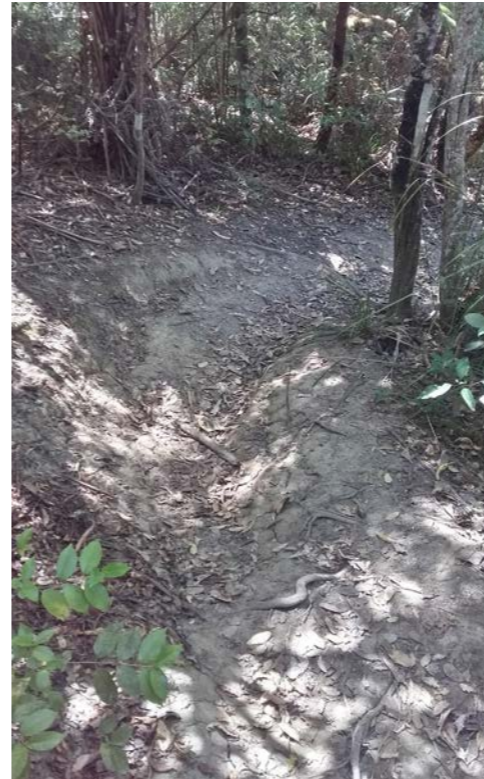
Washed out gravel path and blocked drain
