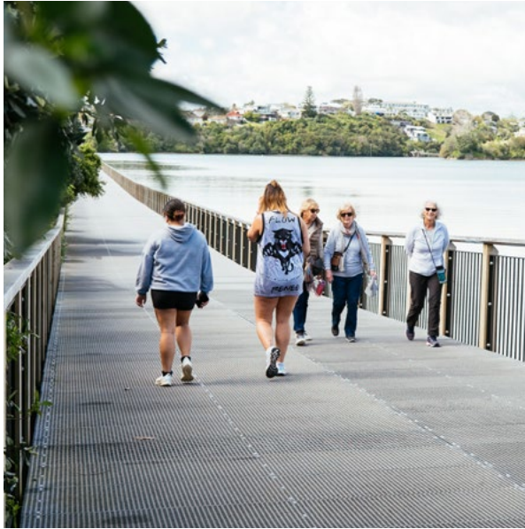
Section 3 of the Glen Innes to Tāmaki Drive Shared Path across Ōrākei Basin.
