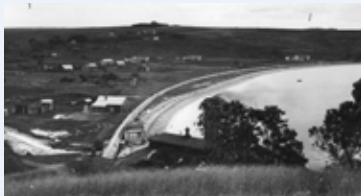
Ōkahu (Matamomoe) showing the sewer pipe which separated the village from the beach, 1921.
