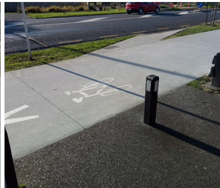
Photo 5: Mt Roskill War Memorial Park colour and texture contrasted delineation between public and park shared paths.
