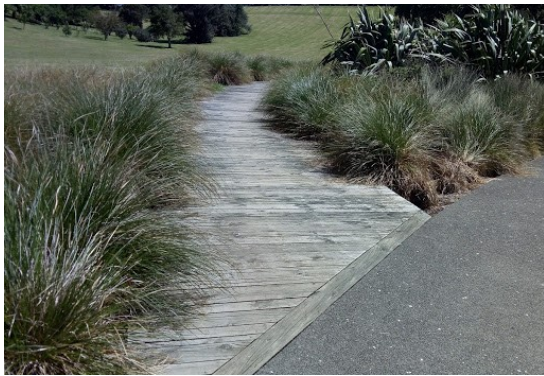
Photo 4: Monte Cecilia Park contrasted texture delineation between footpath and boardwalk.
