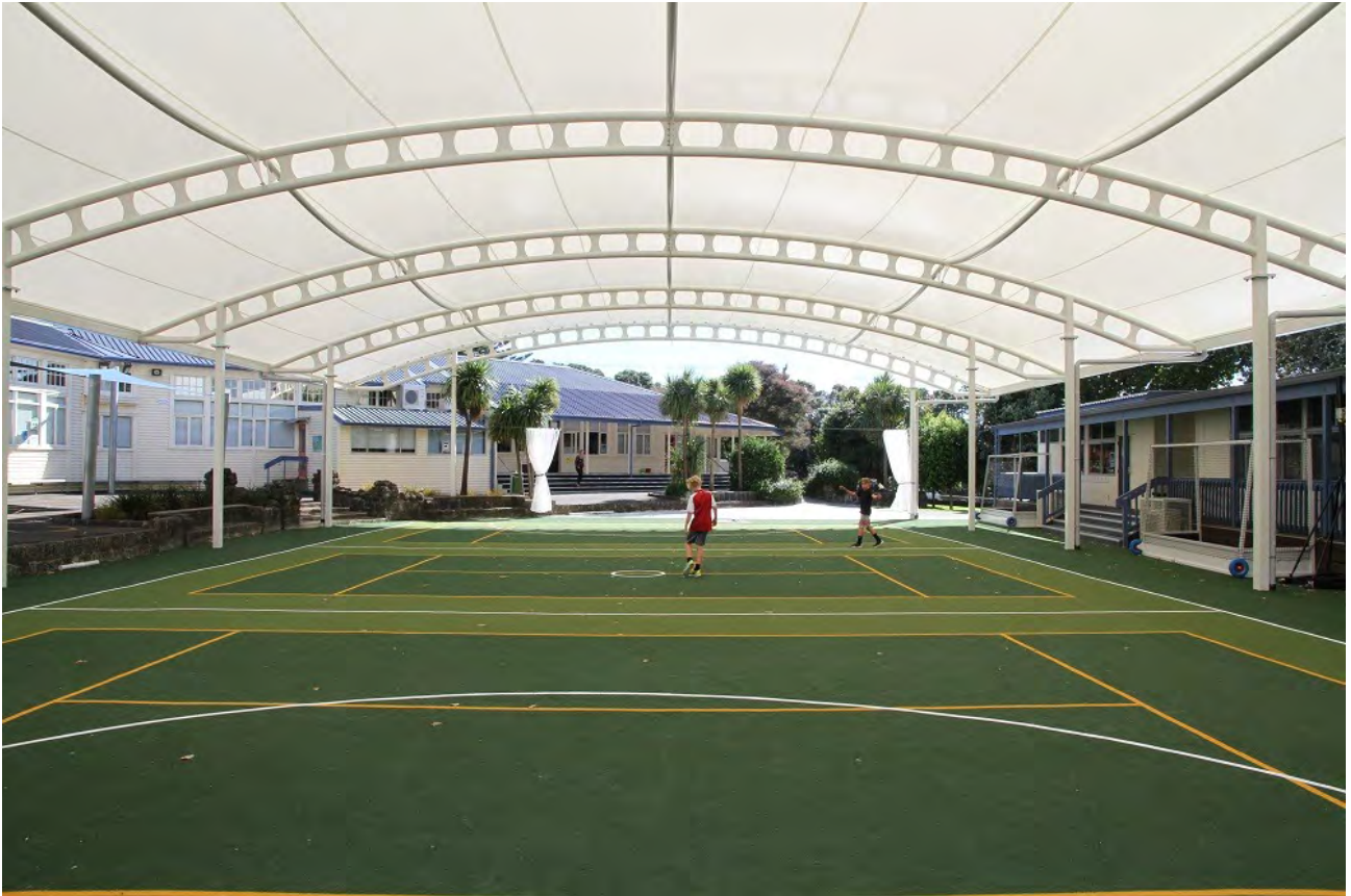
Photograph 9: Shade/shelter structure at Three Kings School, Puketāpapa
