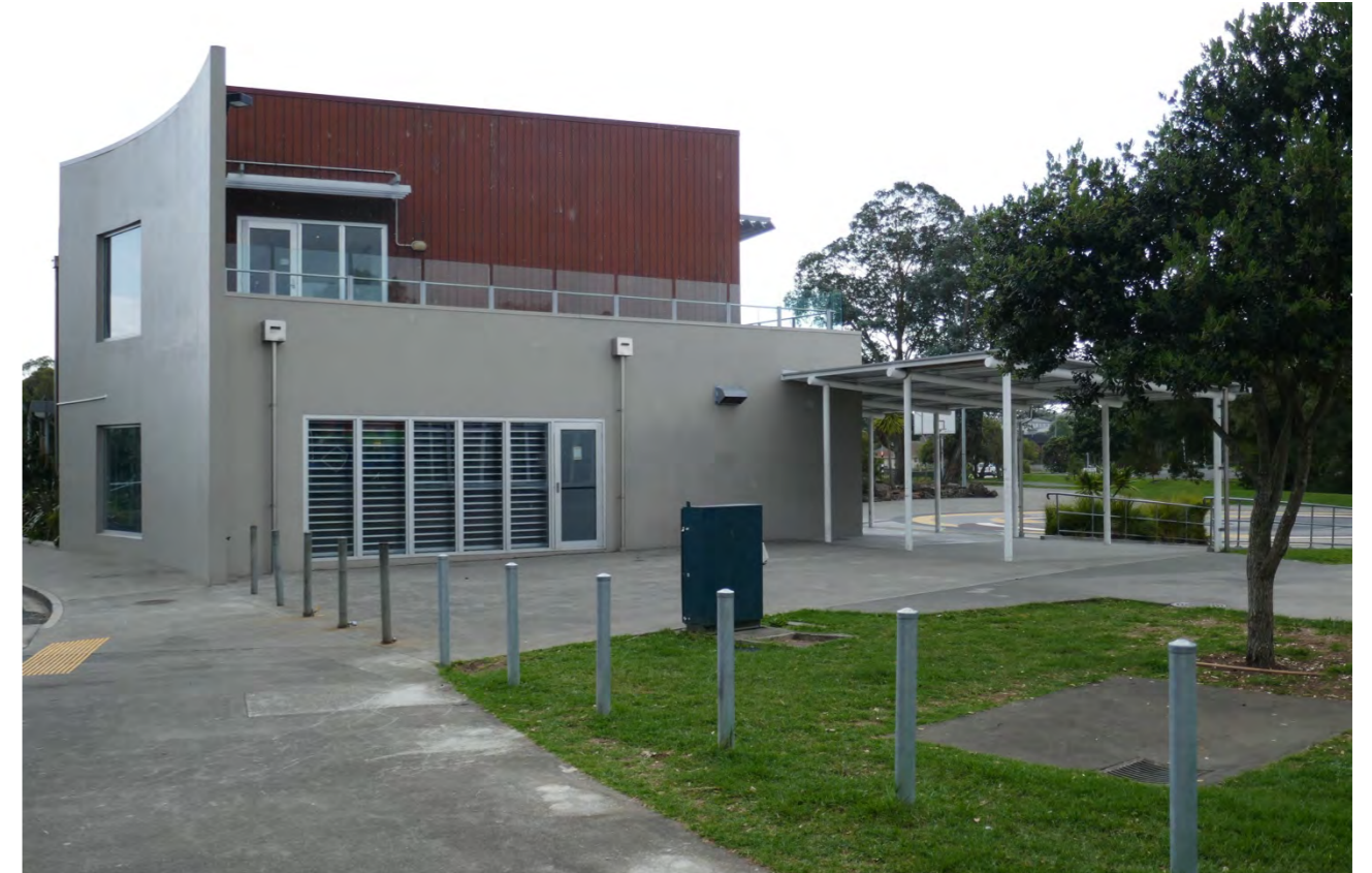
Paved area east of community centre, War Memorial Park
