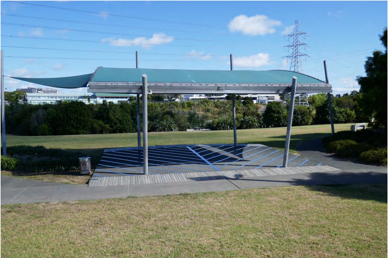
Photograph 3: Shade/shelter/stage structure at Olympic Park, New Lynn
