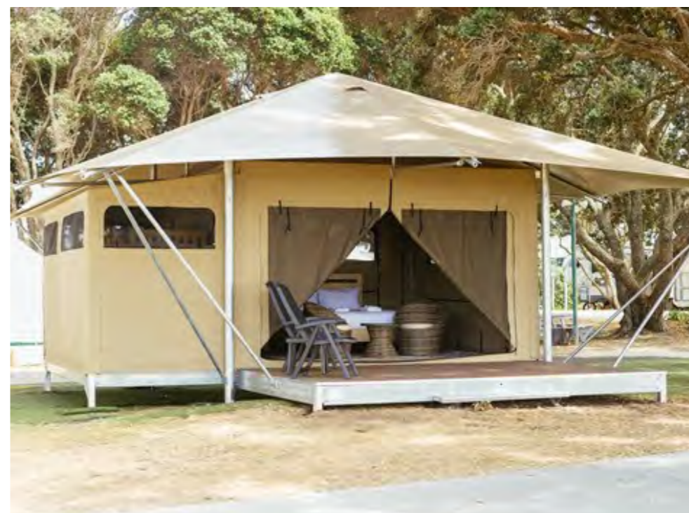
Auckland Council eco-structure for glamping, Orewa
