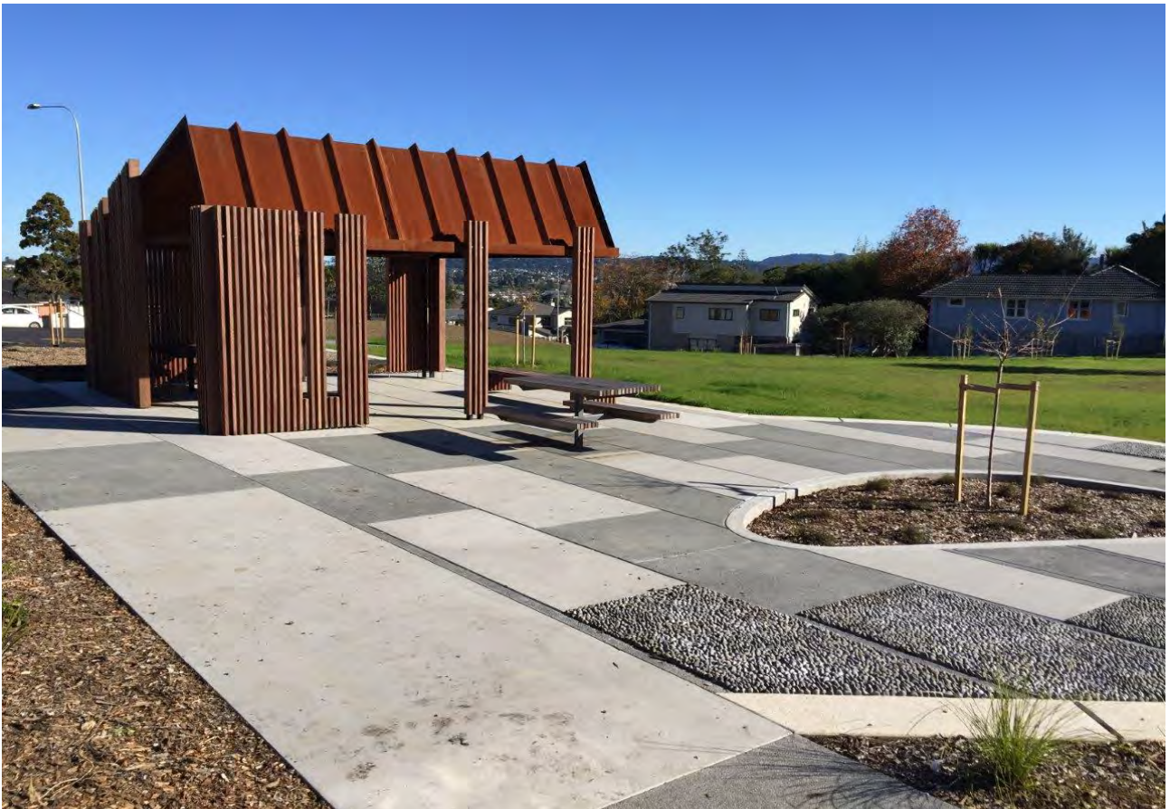
Photograph 4: Shade/shelter structure at Te Kotuitanga Park, New Windsor
