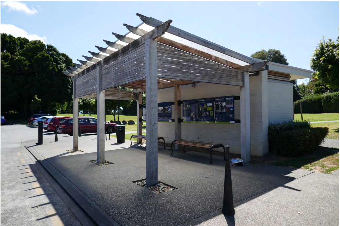
Photograph 1: Shade/shelter structure at Monte Cecilia Park
