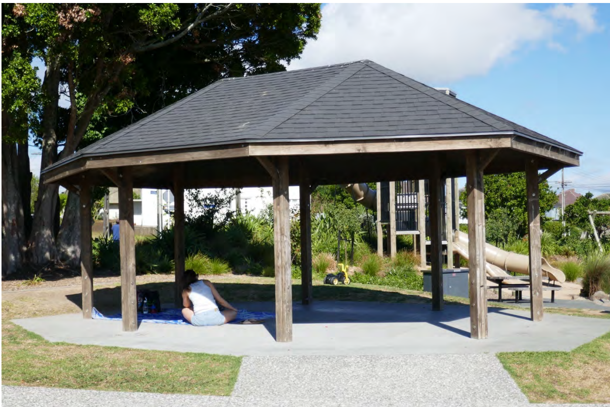
Photograph 6: Traditional wooden shade/shelter structure at Waterview Park, Waterview
