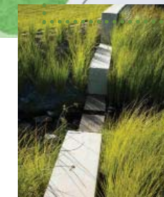
L: Grass bunting to along edge of grass slope to restrict flow of stormwater and damage to planting on lower slopes
