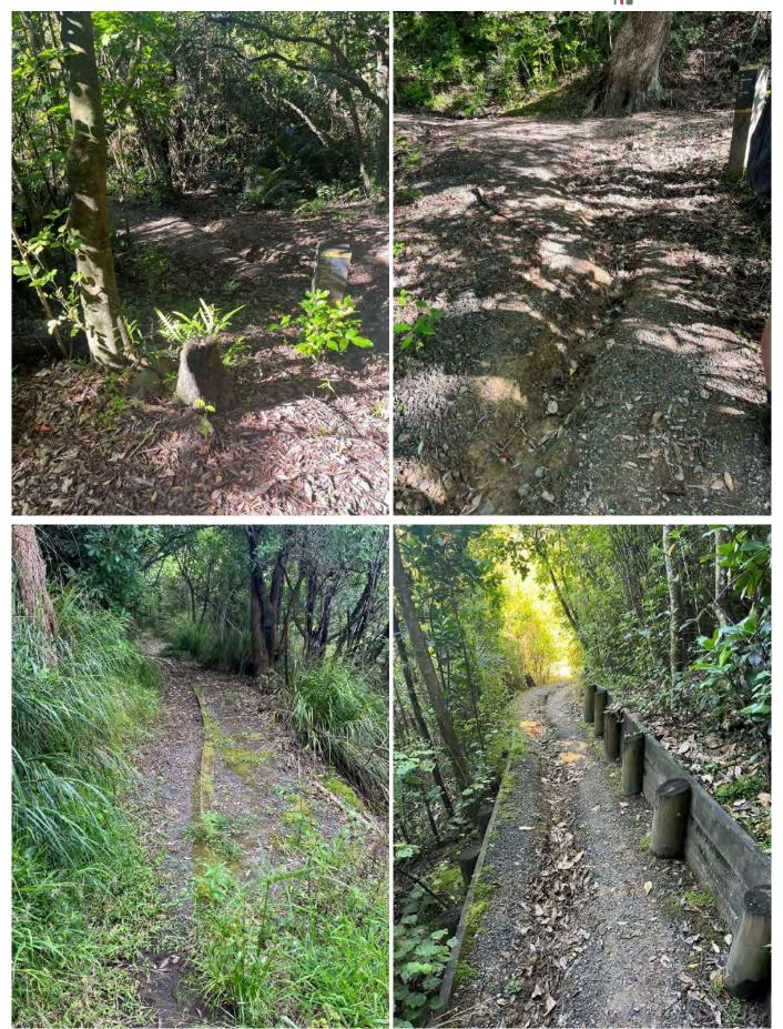
Figure 17: Captains Bush - Aggregate track scour
