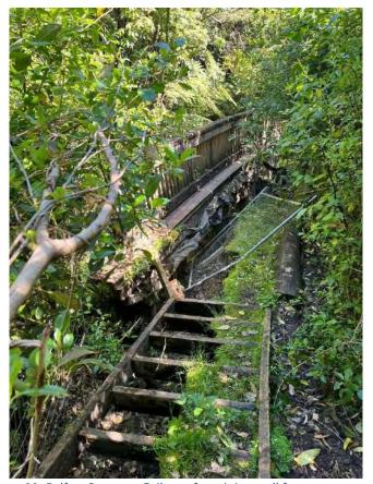
Figure 29: Belfast Reserve - Failure of retaining wall from stream scour
