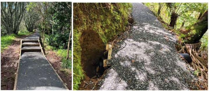
Figure 33: Edged aggregate track and boxed steps (left), culvert (right)
