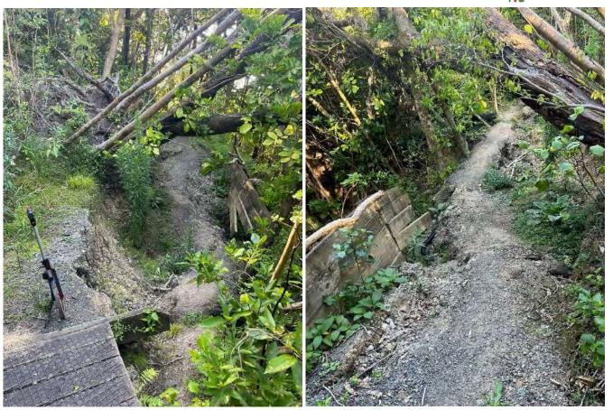
Figure 14: Captains Bush - Slip and failed retaining wall
