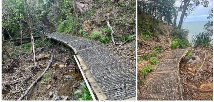
Figure 3: Manukau Domain - lower slip on boardwalk structure
