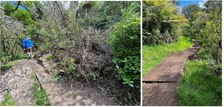
Figure 9: Wattle Bay - Slip debris on concrete path (left); ground movement resulting in failed concrete path (right)
