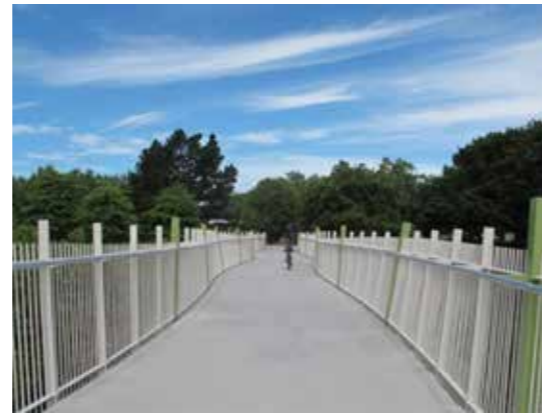
Waterview Path over Te Auaunga Awa (Oakley Creek) to Unitec
