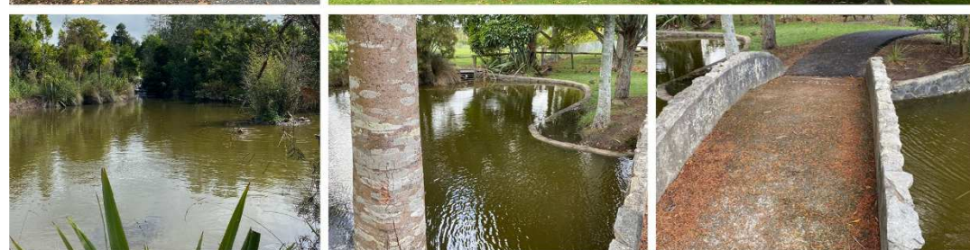
Stormwater pond adjacent northern fields
