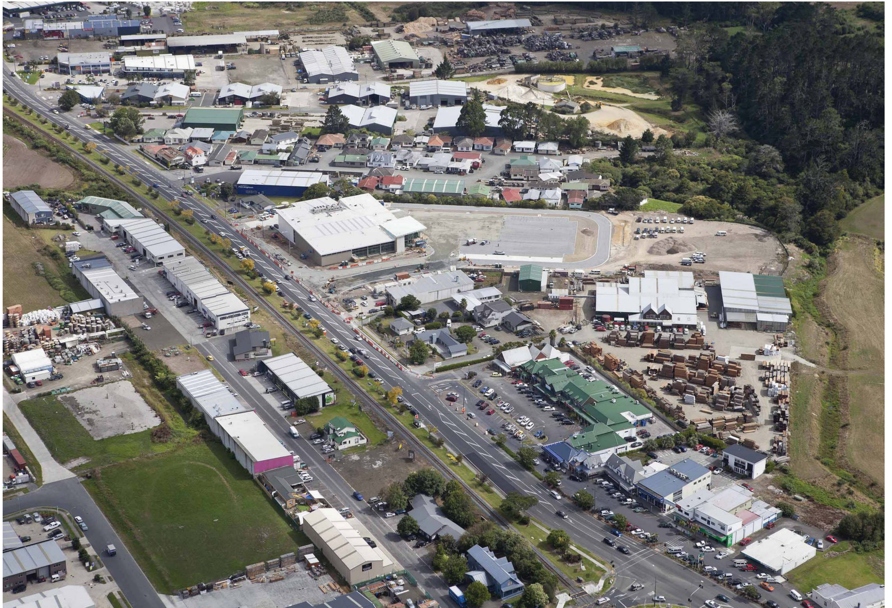
Looking down on Kumeu Town Centre, the New World Supermarket under construction centre of image.
