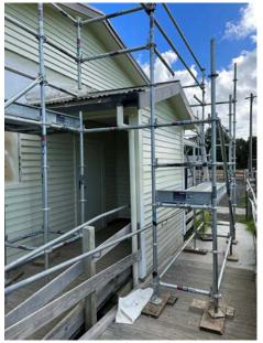
Above: Front of hall, new cladding being painted, minor roofing repairs underway.
