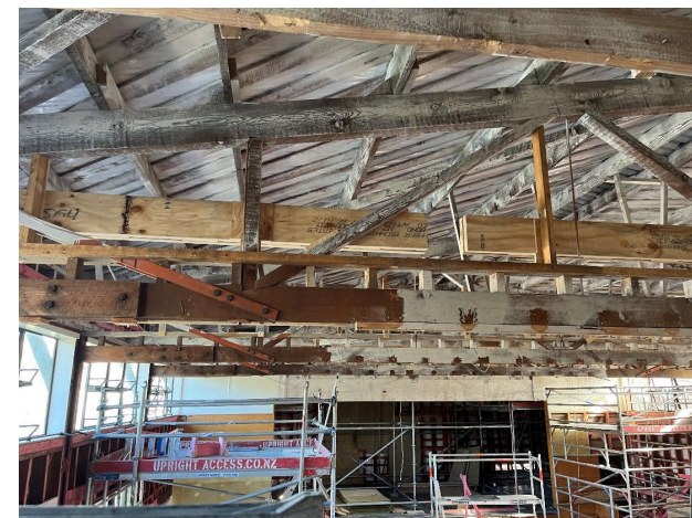
Inside of hall with ceiling removed
