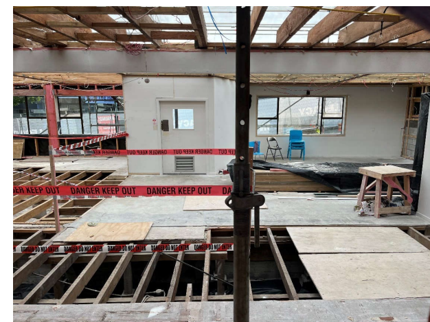
Inside of RSA with roof and floor partially removed
