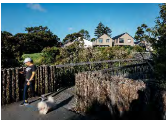
East Sunderland Bridge, Hobsonville
