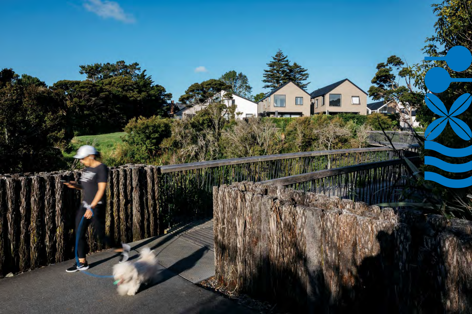
East Sunderland Bridge, Hobsonville
