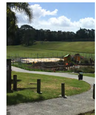
Current renewal work
