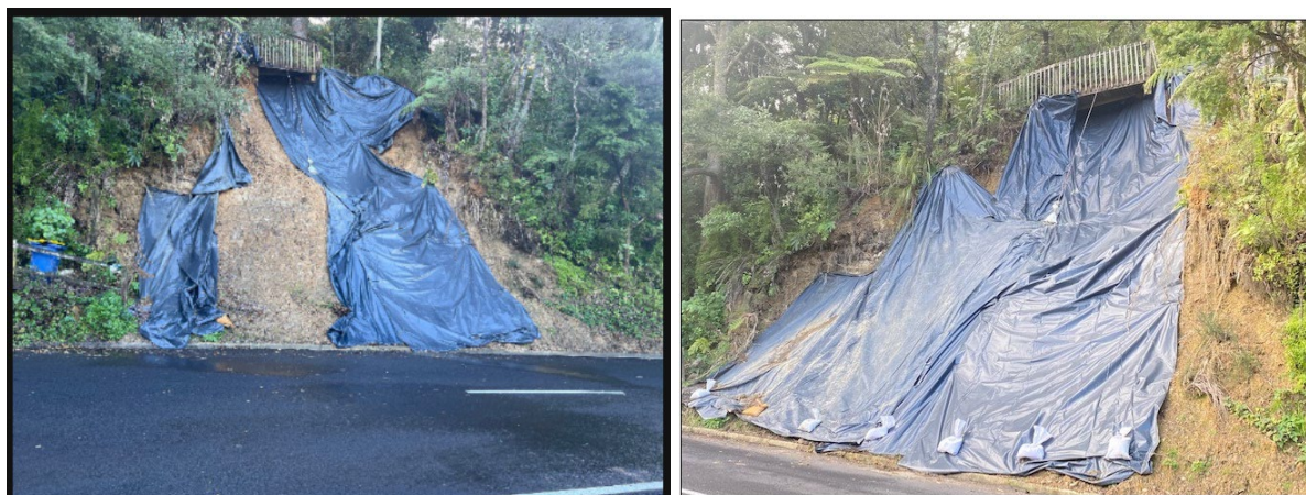
Warner Park Rd polythene repair.
