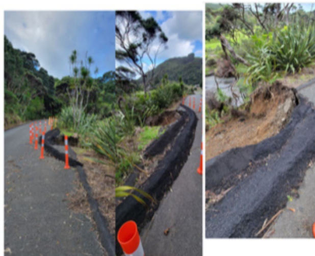
Tasman View Rd- new polythene cover installed.
