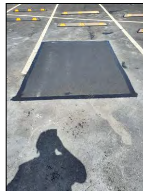
Asphalt burning - remediated
