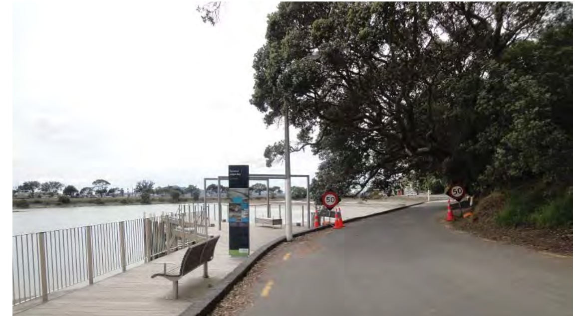
Judges Bay Road - connection to Parnell Baths (showing boardwalk section)
