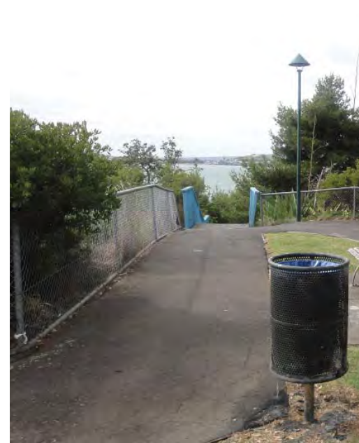
Current staircase down headland
