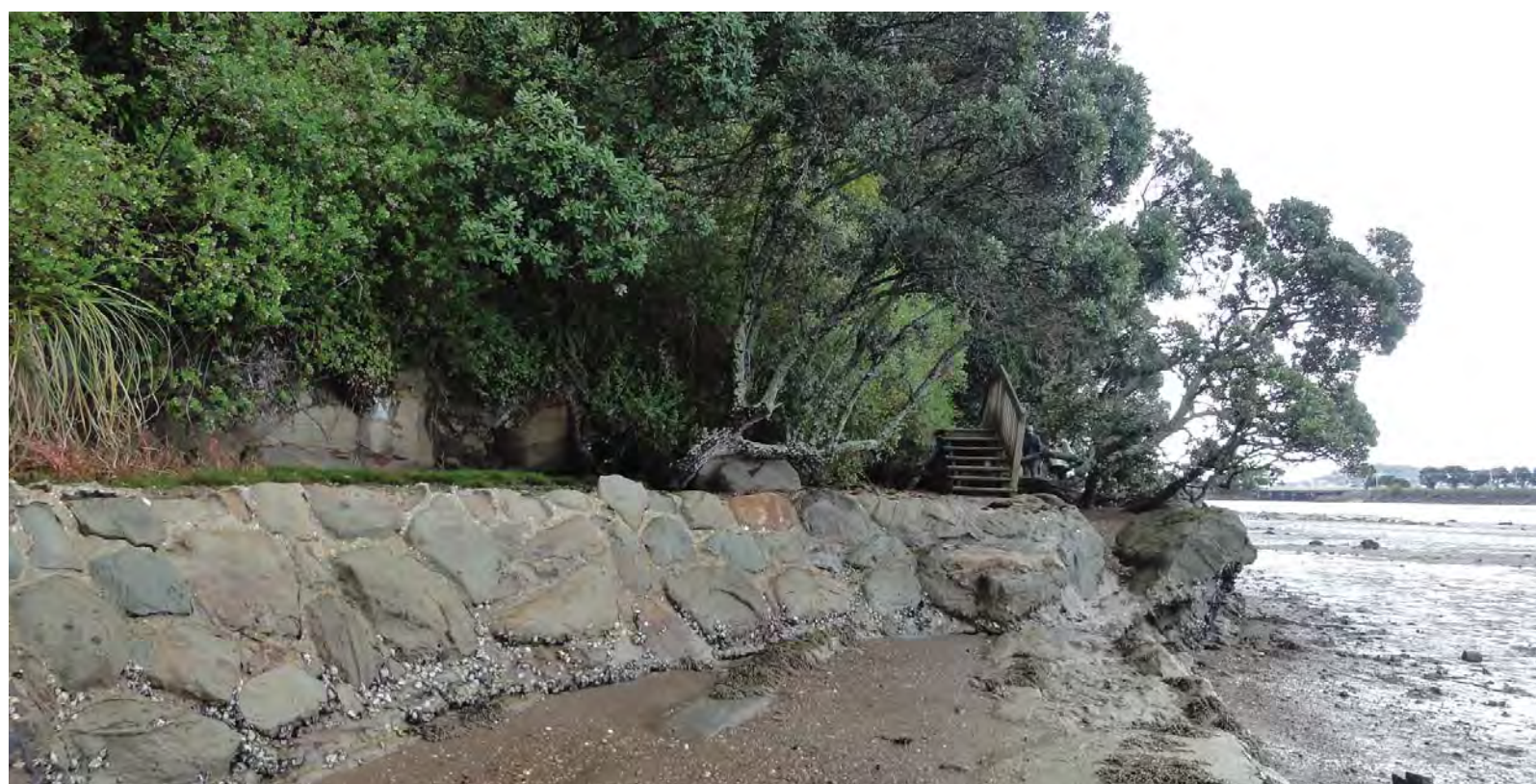
Figure 4: Hobson Bay Walkway - showing mudcrete and stone wall. 2014.
