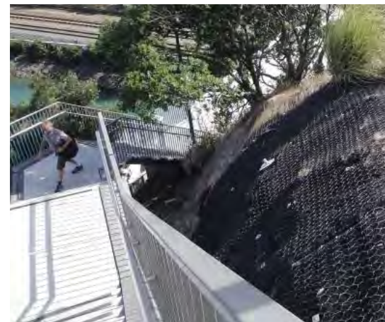
New staircase and recent bank stabilisation
