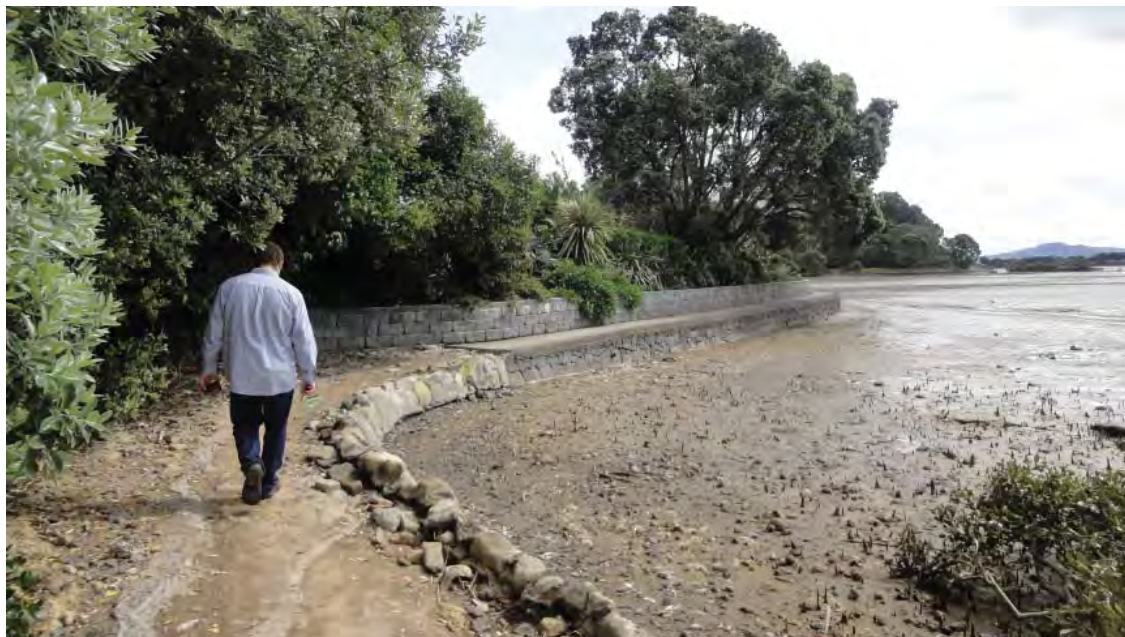
Hobson Bay Walkway - location opposite Tohunga Crescent
