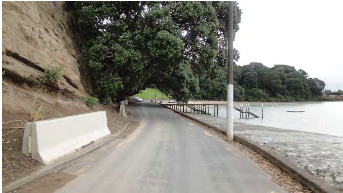
Judges Bay Road - connection to Parnell Baths - no designated path for pedestrians
