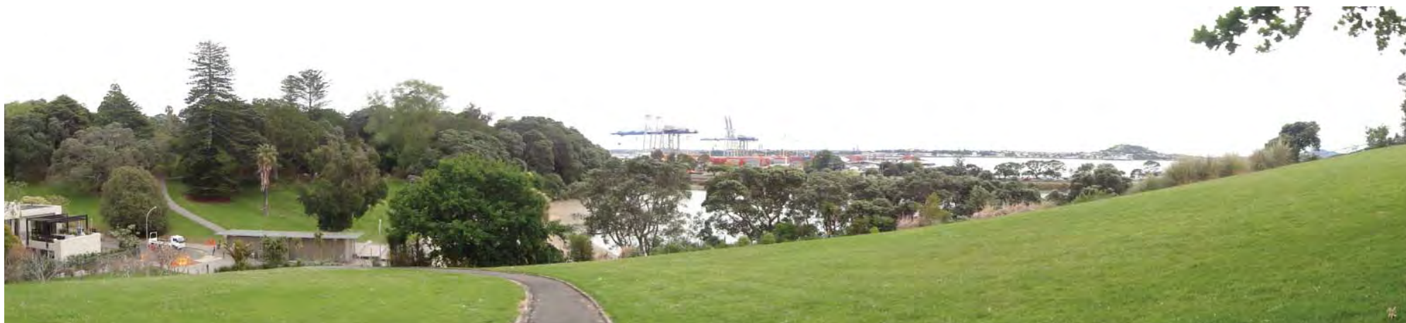
View looking north to Ports of Auckland over Judges Bay from Judges Bay Reserve
