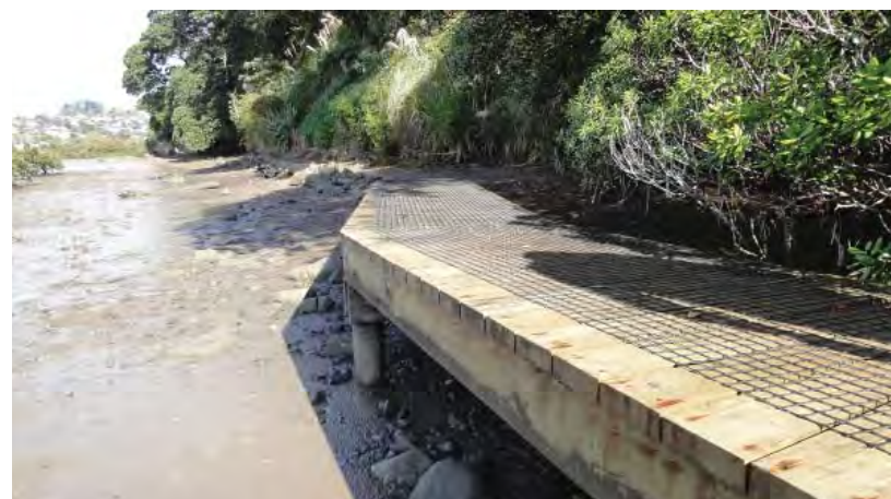
Hobson Bay Walkway - section of boardwalk
