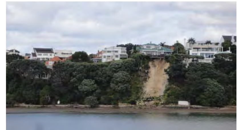
View from Tāmaki Drive to the slip
