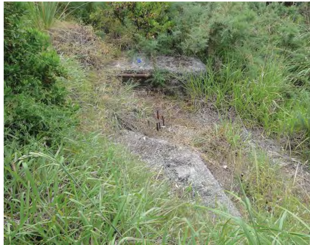
Figure 15. Part of the eastern gun emplacement as is visible today.
