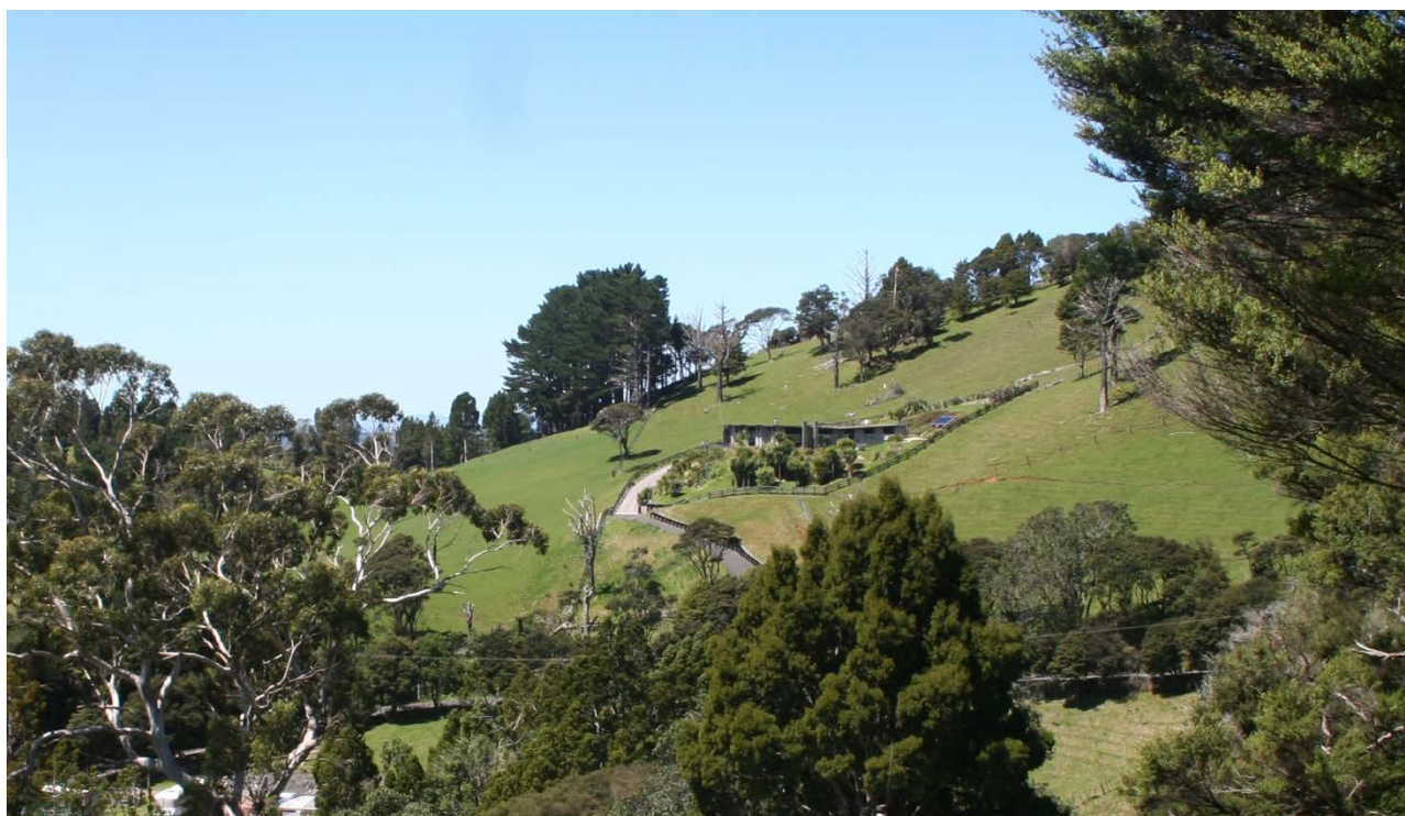
A new house in Little Huia was under construction in 2012. The form, height, materials and colour of the building and the associated garden development all ensure that this new house sits comfortably within the landscape unit and does not undermine the heritage features (2017). (Source: Melean Absolum)
