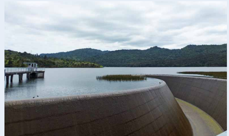
Lower Nihotupu Dam
