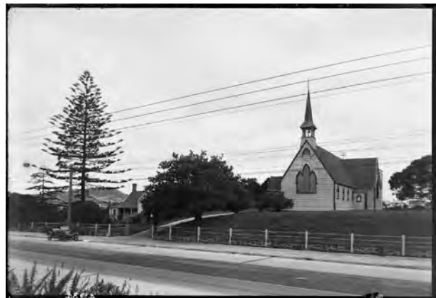
Figure 72. Looking south from New North Road towards St Luke's Church, Mount Albert (1934).
