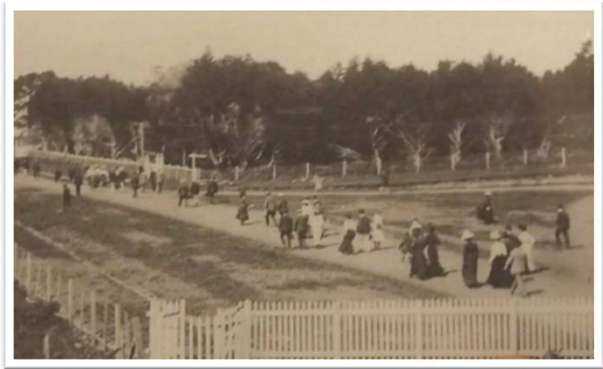
Figure 11. 1910 view of John Fairburn grounds opposite the Otahuhu railway station corner of Walmsley and Sale Yard Road (2012). The vegetation was grown to form a noise (trains and industry) and industrial pollution buffer.
