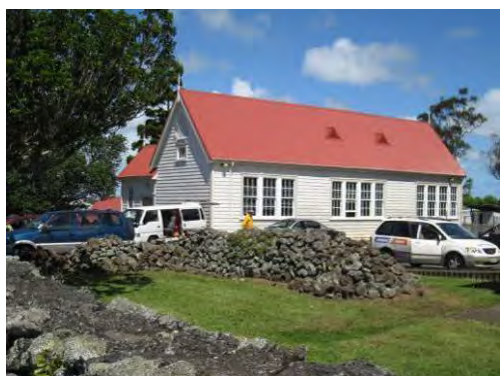
Figure 13: Old school house (top) and hall on Kirkbride Road, Mangere Central.
