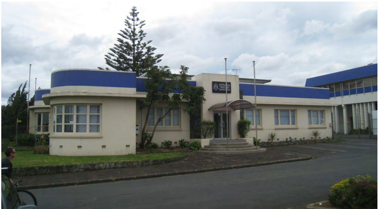
Aotearoa Technical Institute at 14 Walmsley Road, Otahuhu Photograph AJ Matthews, November 2012.
