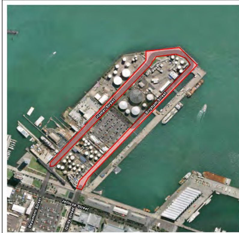
Roadside parking near Wynyard Tank Farm Brigham Street and Hamer Street, Wynyard Quarter
