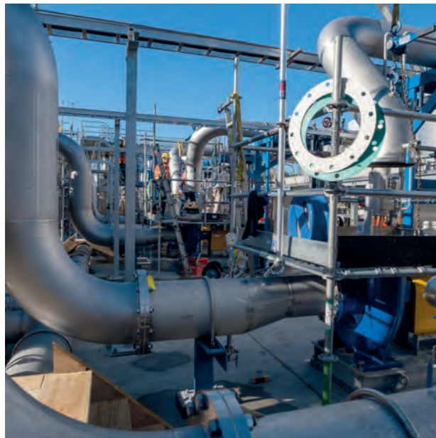
The new water treatment plant in Tuakau
