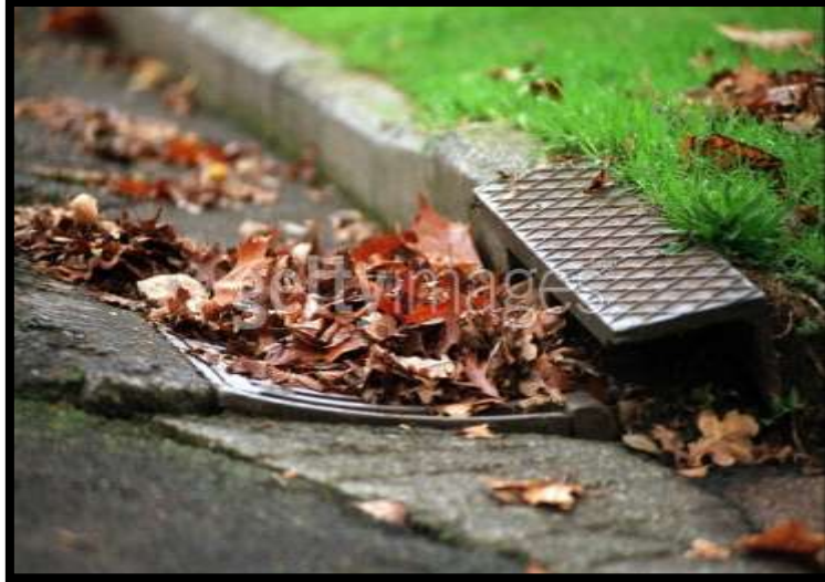
Fig 4: Blocked drains in Ponsonby - Franklin Road (note: permission to be sourced from photographer)
