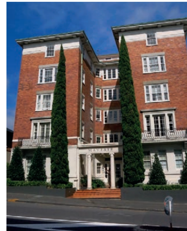
Mayfair apartment building, Parnell Road.
