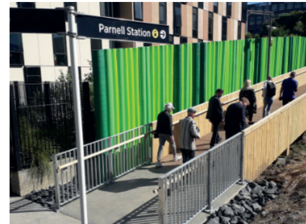
Access to Parnell train station from Nicholls Lane extension (formerly Carlaw Park).
