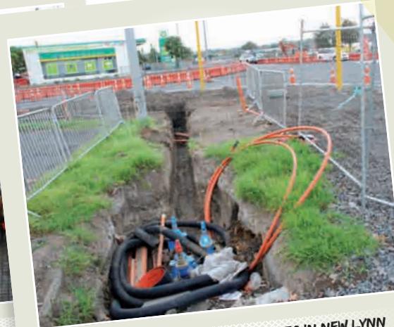
INSTALLATION OF FIBRE OPTIC CABLES IN NEW LYNN STREETS - 2010
