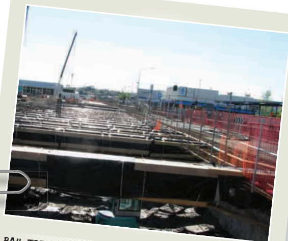
RAIL TRENCH CONSTRUCTION
