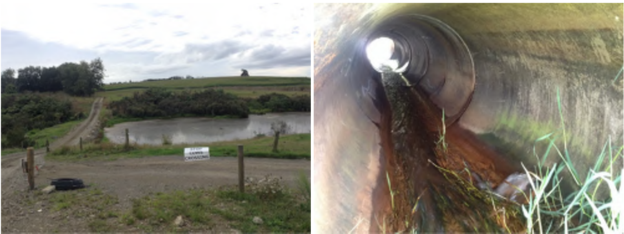
Figure 27: Culvert at online dam (NGAF_114)
