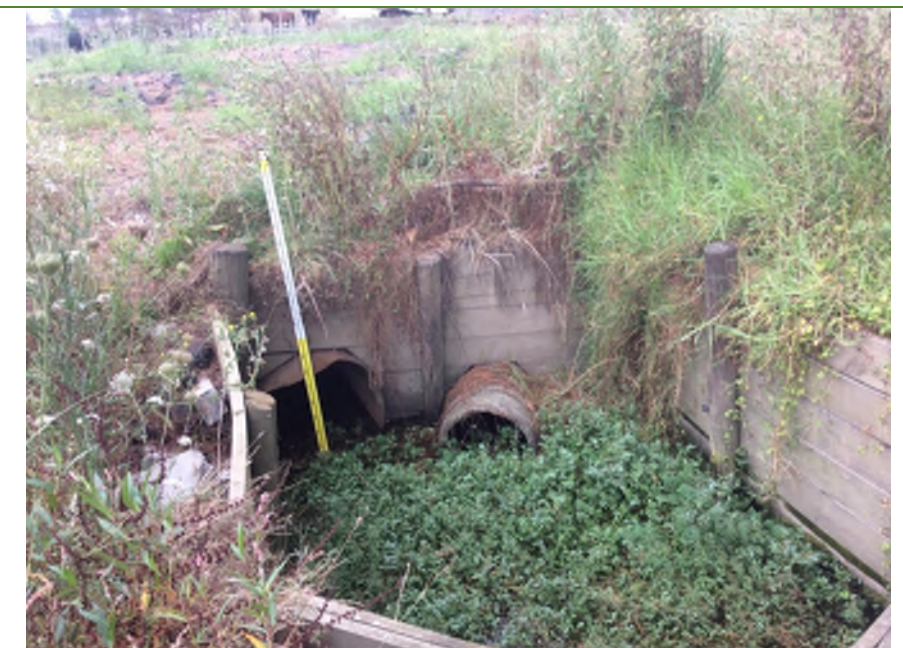
Two concrete and cast-iron pipes at culvert outlet
