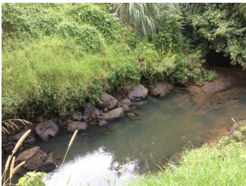
Figure 29: Rock bank lining along NGA_MAIN_2, which appeared safe and had easy access.
