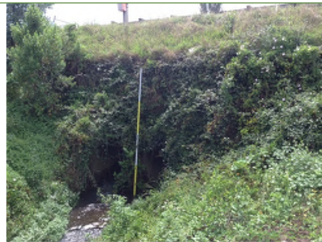
Culvert outfall under motorway (NGAR_006)
