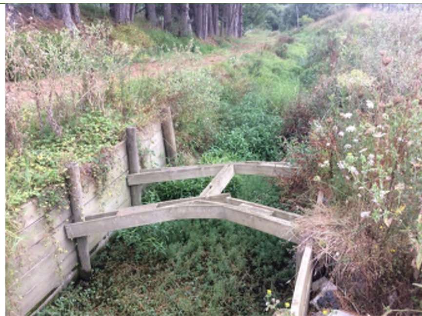
5 m length timber lining with cross beam reinforcing at culvert outlet
