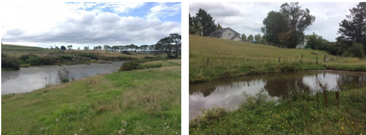
Figure 19: Large online dam at NGAWEST_6 (left) and typical farm pond, NGA_TRIB6_1 (right)
