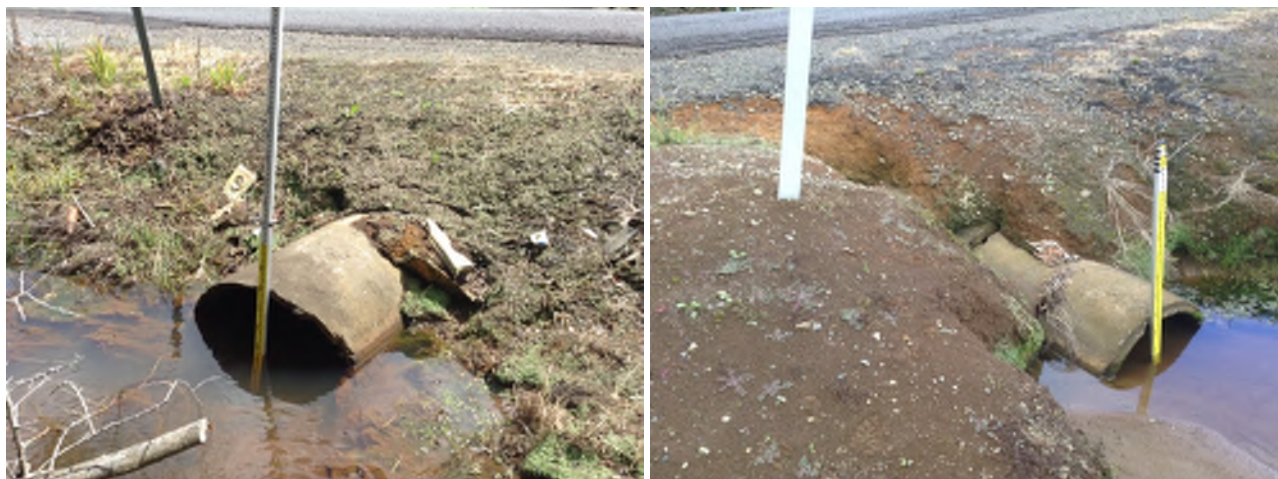
Figure 24: Left - Inlet (NGAR_047) and Right - outlet (NGAR_067) at Beaver Rd
