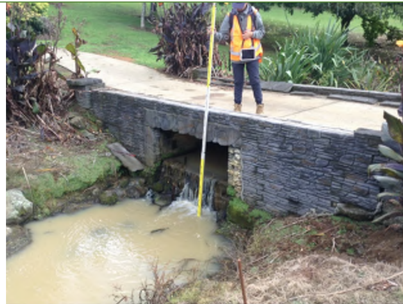
Box culvert at golf course at Ingram Rd (NGAF_033)
