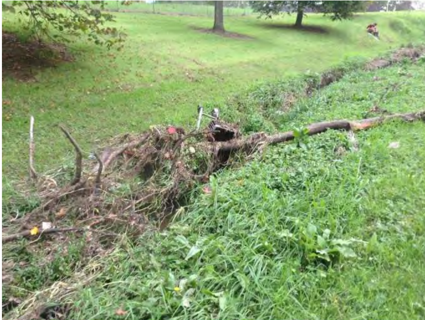
Figure 36: Debris jam obstructing flood flow caused by a shopping trolley on SLI_MAIN_31 at Keri Downs Park
