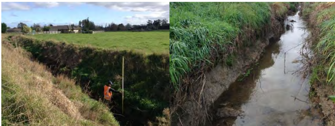
Figure 6: Representative reach of the main channel of WAI_TRIB2 with a close up of side cutting.
