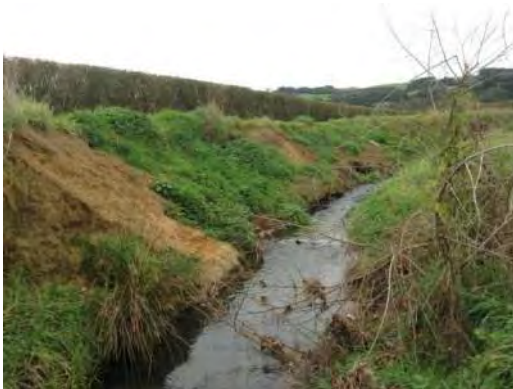
The true right bank on WAI_MAIN_12 has been widened and regraded. Pasture grasses on both banks.
