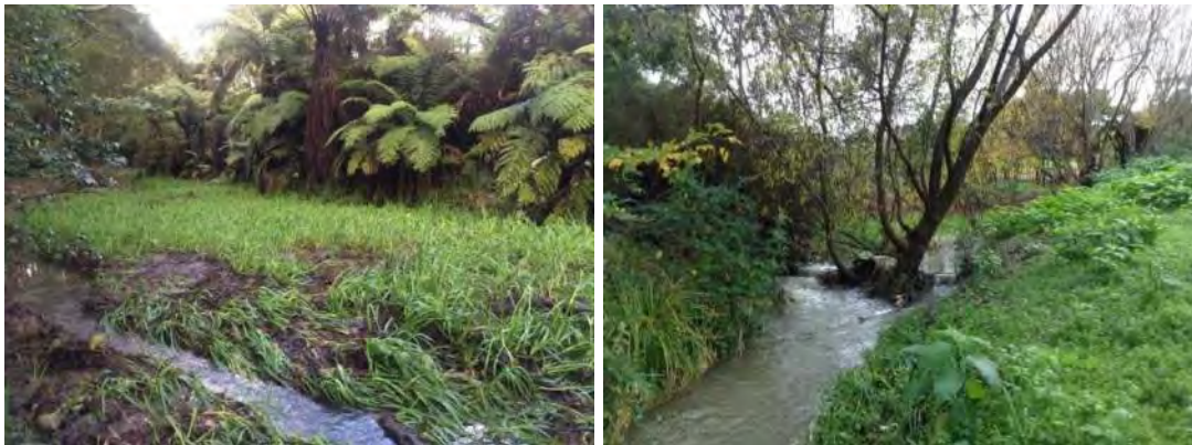
Upper Croskery Drain Catchment Flood Detention Dams Project 15
