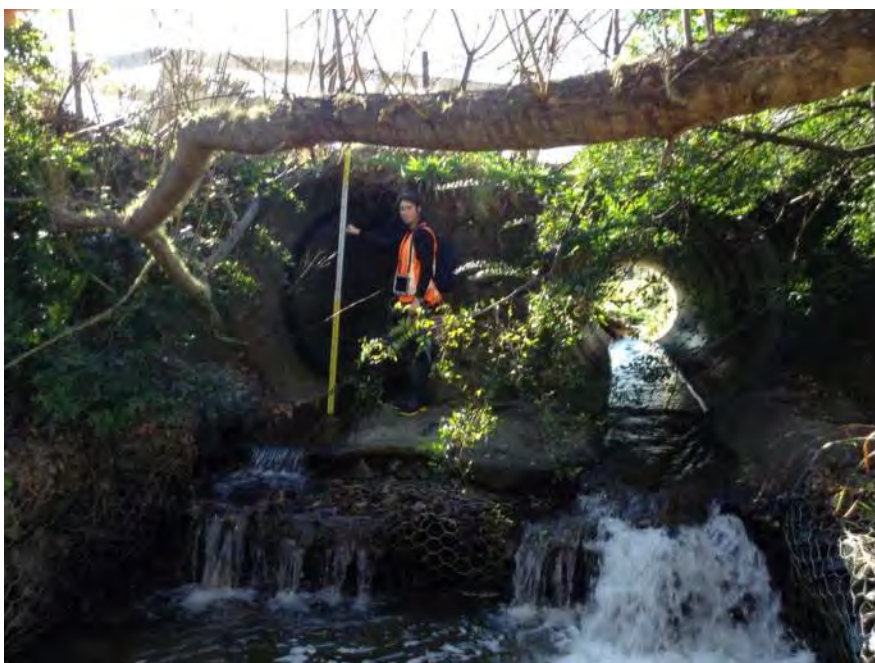
Figure 20: Concrete apron at the outlet (UNK_237) on Symonds Stream (SYM_MAIN_19).
