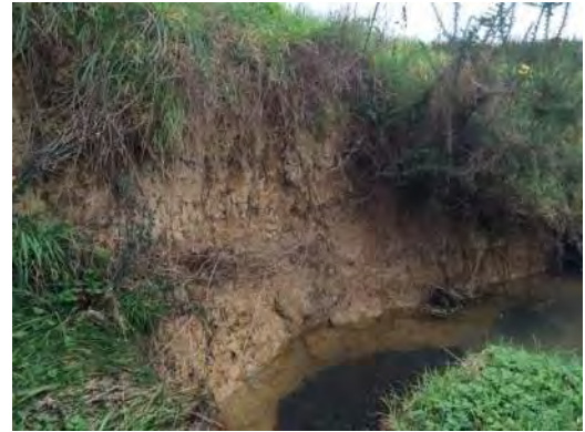
Erosion hotspot on true left bank
