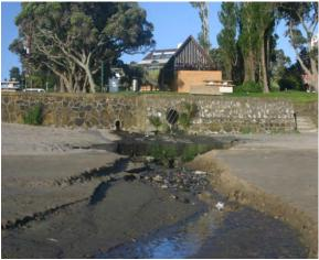
Figure 5.15 Coastal outfalls with erosion, Takapuna
