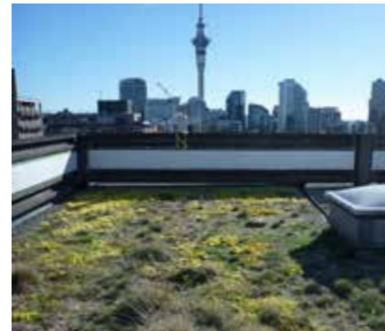
The University of Auckland green roof
