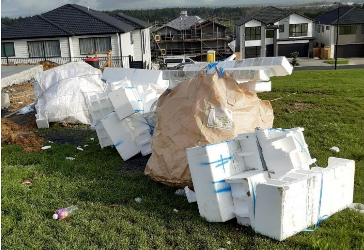
Figure 3 Improperly contained EPS on-site allows beads or snow to escape.
