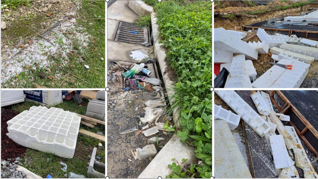
Figure 4 EPS snow/bead contamination after hand-sawing on-site and general litter blocking drains at the Flatbush residential development in South Auckland (photo courtesy of Auckland Council Environmental services)
