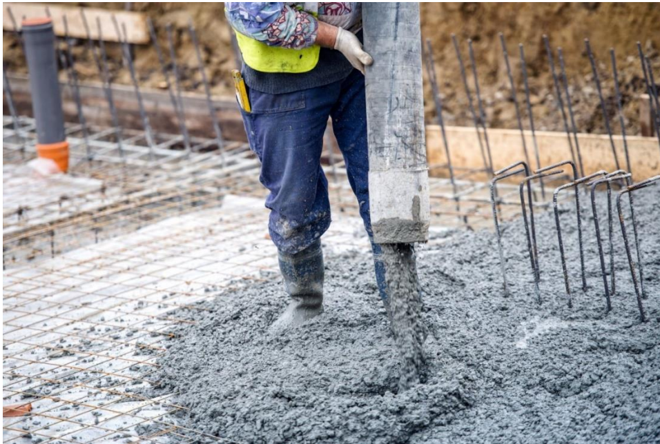
Figure 2 EPS slabs with rebar framing for load bearing and rigidity with concrete poured over bonding the materials.
