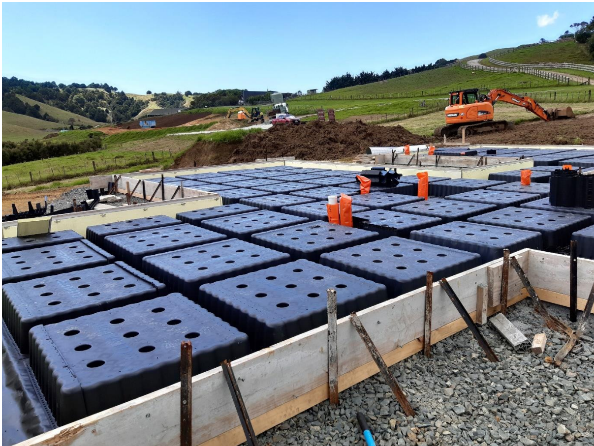
Figure 8 ClevaPod system enabling the separation of reusable plastics from concrete at end of life.
