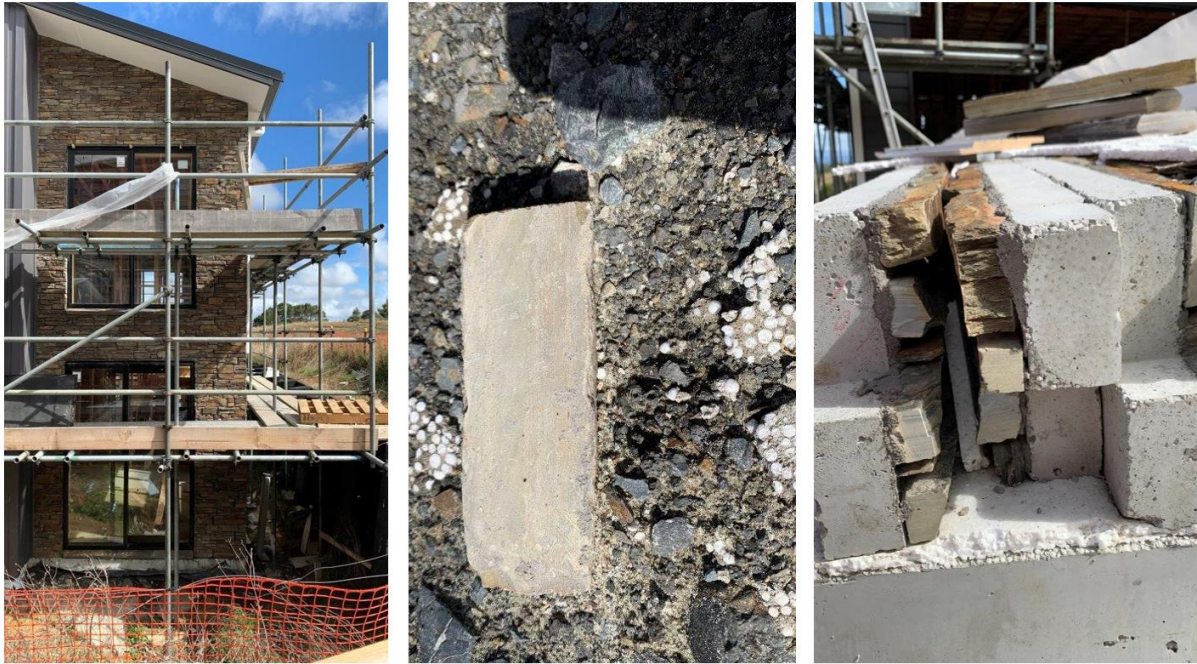
Figure 1 Examples of the use of EPS in stone facades and EPS beads having escaped into the environment during cutting.
