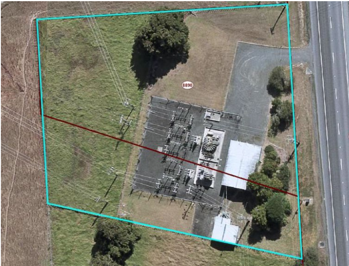
Figure 3: Satellite image of switchyard, showing the designation and property boundaries.
