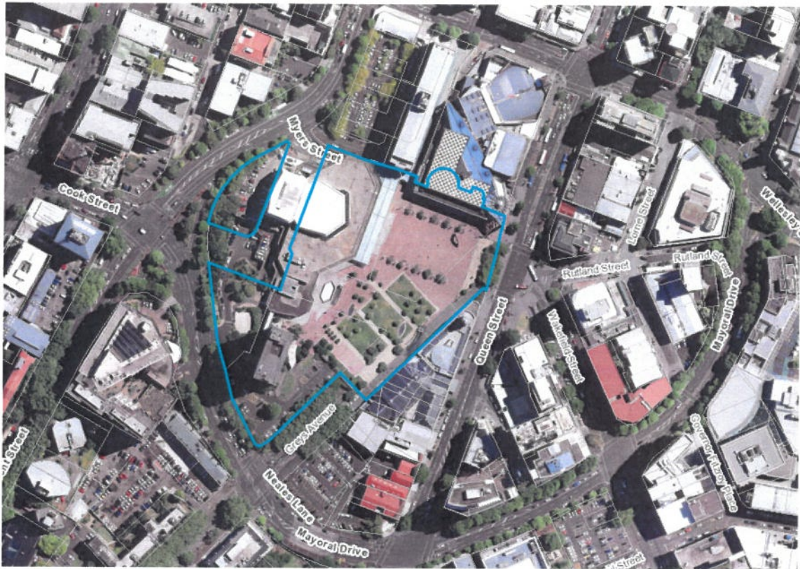
Figure 1: Aerial photo of subject site, 299 Queen Street, Auckland Central. Location of the Civic Car Park
