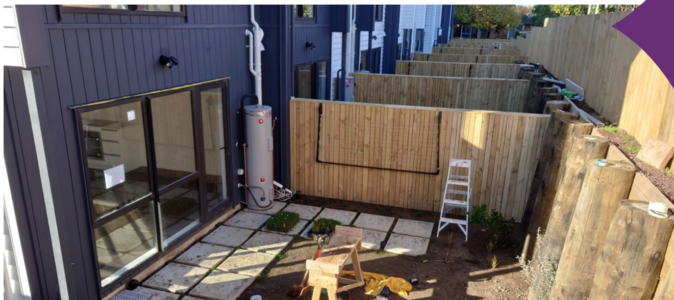
A high retaining wall combined with a fence can reduce daylight and cause shading to indoor and outdoor living spaces.
