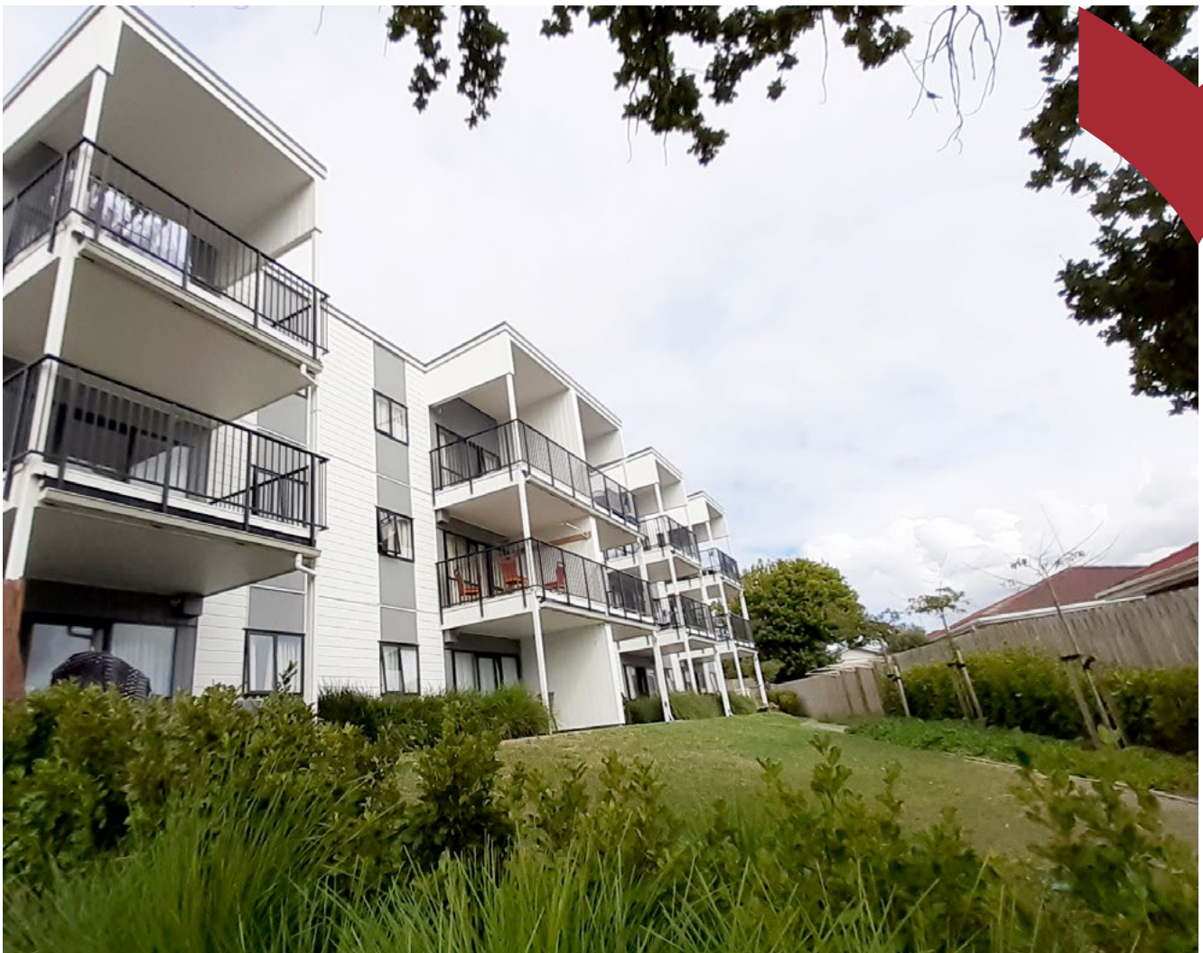
High density apartments within landscaped site minimises adverse dominance and privacy effects on adjacent site.
