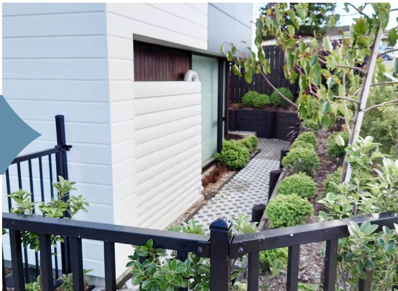
A good example of a narrow rainwater tank integrated with the building and permeable quality landscaping.
