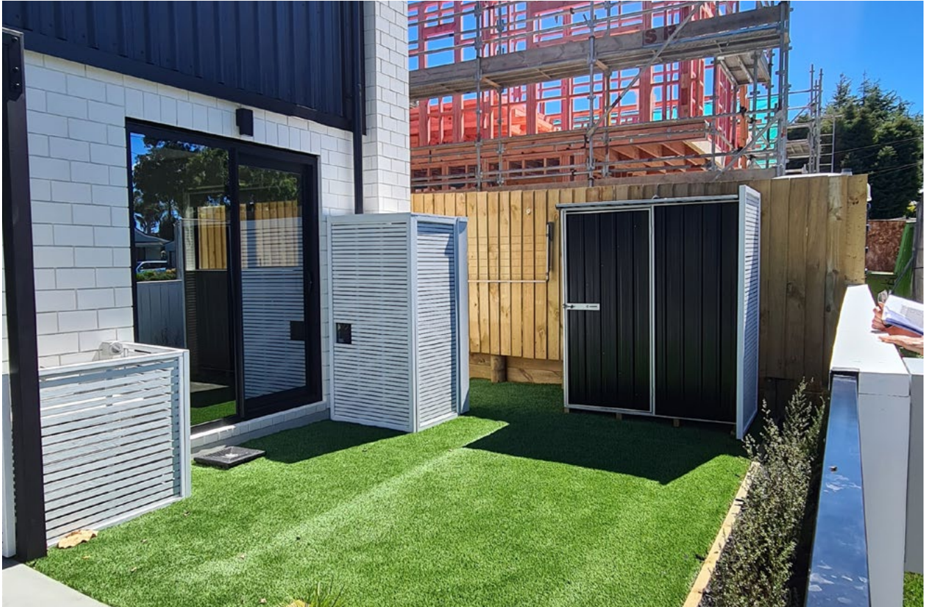
The useable space of the ground floor outdoor living area is reduced by the presence of a heat pump, shed and water tank. In this site, the items are screened.
