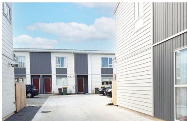
A development with front doors opening directly onto a communal parking area and vehicle manoeuvring space. The designated footpath area (dark grey paving adjacent to the dwelling on left), directs pedestrians into the reversing space of cars en-route to the front doors of dwellings. These are all pedestrian safety concerns – especially for children.
