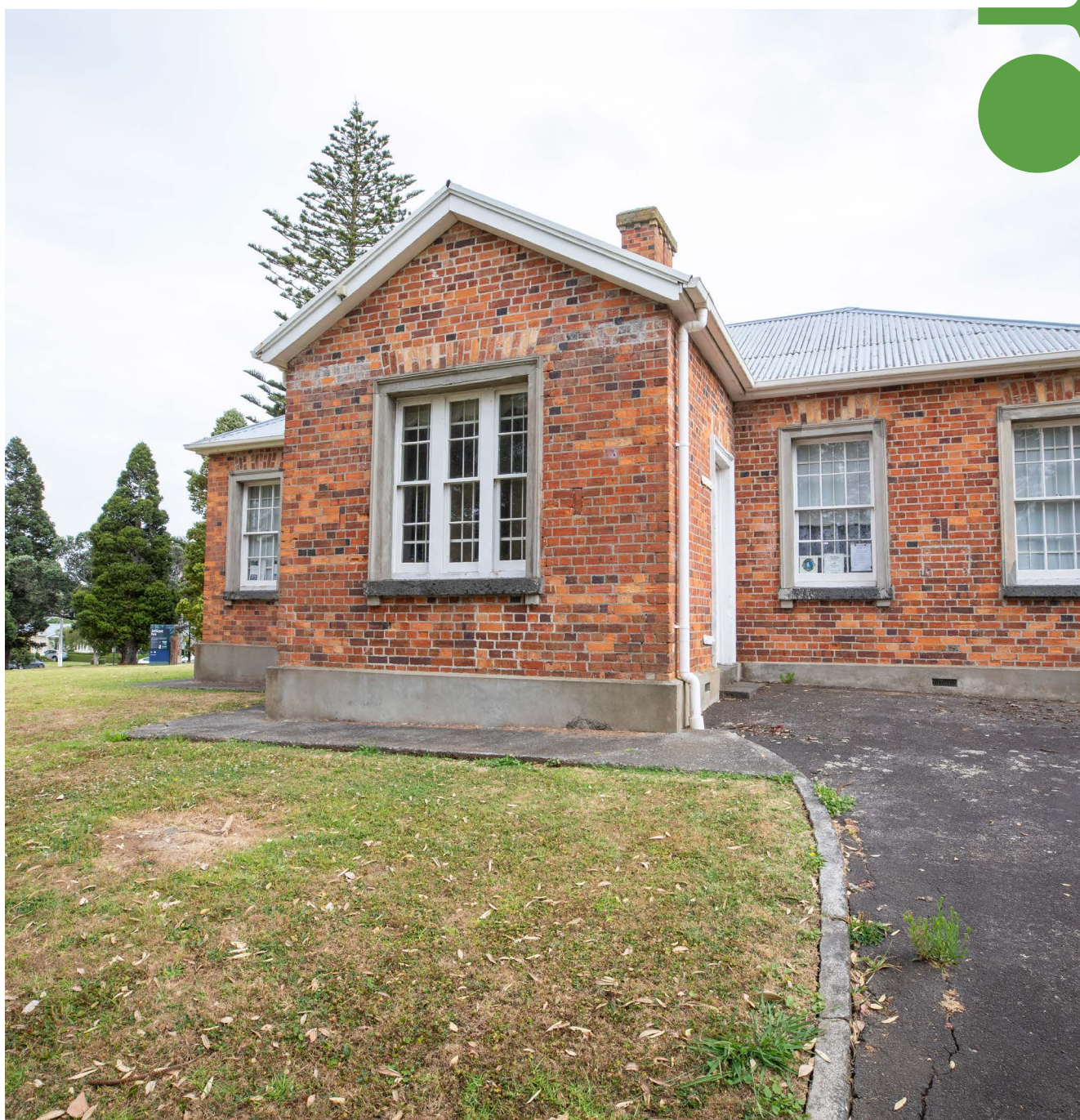
Onehunga Blockhouse (Category A historic heritage place).
