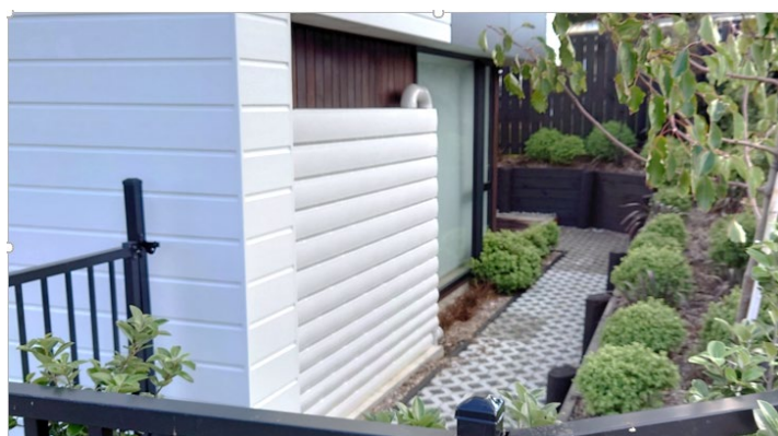
Figure 27. An example of a narrow rainwater tank integrated with the building and permeable landscaping.
