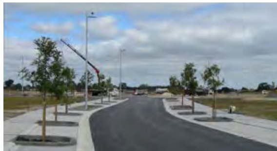
Example of minor street under construction (Buckley Precinct)
