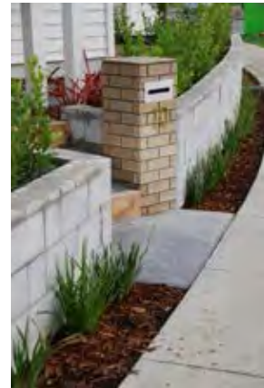
Concrete block retaining wall to front boundary with planting to screen.
