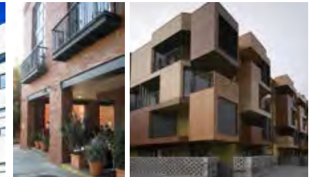
Building line variation
