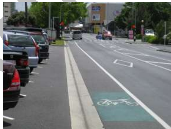
Figure 8: Cycle lane next to angled parking (Rainside Ave Akl) (substandard)
