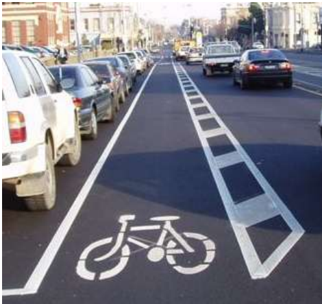
Figure 11 : Buffered cycle lane Melbourne – but note insufficient width to parked cars
