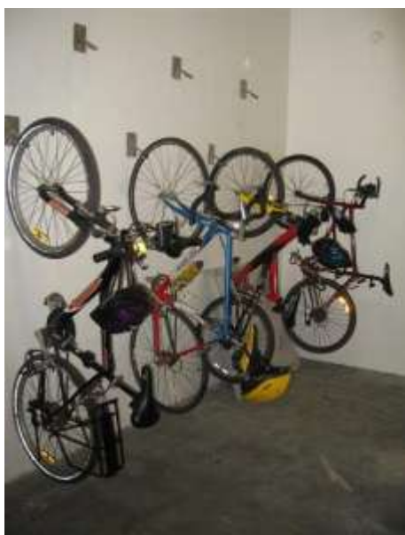
Figure 59: Wall hanging cycle racks (S Mills)
