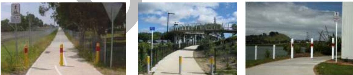
Figure 36: Examples of Bollards on shared path from left to right: Austroads (2009m), SH 20 cycleway near Keith Hay Park (Akl), Waikaraka cycleway (Akl)
