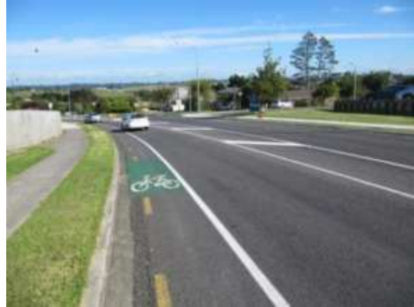
Figure 3: Cycle lane with colour highlight, white cycle logo and “no stopping” lines, Auckland
