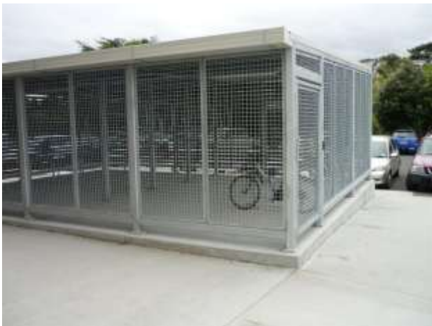
Photograph 2: Cycle Parking Cage – Middlemore Hospital (K Hancock)
