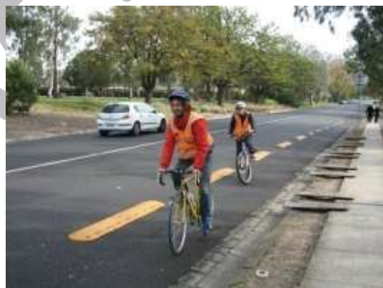
Figure 4 and 5 : Rubber kerb example (Sources: Riley left, Vic Roads right)
