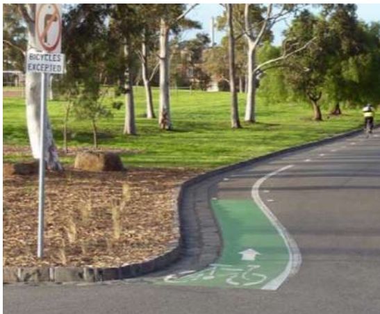
Figure 17: Contra-flow lane on left kerb (one way general traffic approaching viewpoint)
