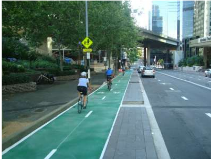
Figure 15: Two-way protected cycle facility with parallel parking (Sydney)
