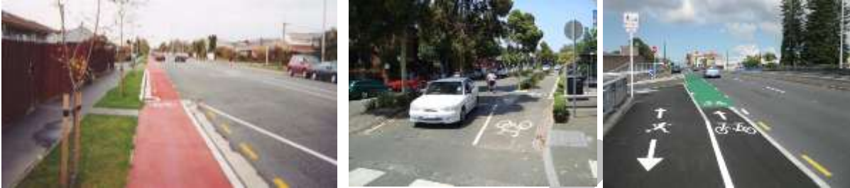
Figure 24: Examples of cycle path converting to cycle lane to give cyclists priority through intersection (from left to right; Christchurch, Melbourne, Akl Ian McKinnon Drive)
