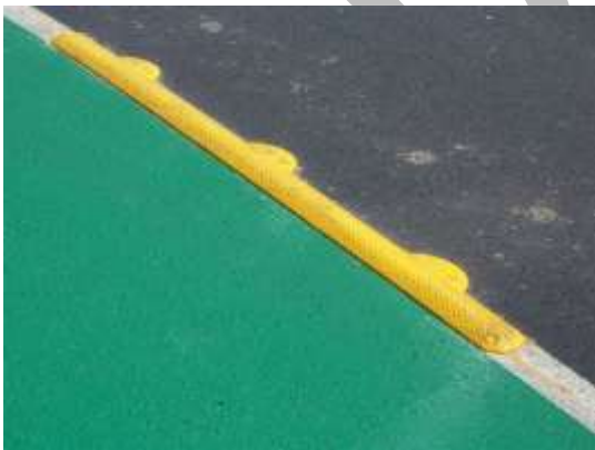
Figure 4 and 5 : Rubber kerb example (Sources: Riley left, Vic Roads right)
