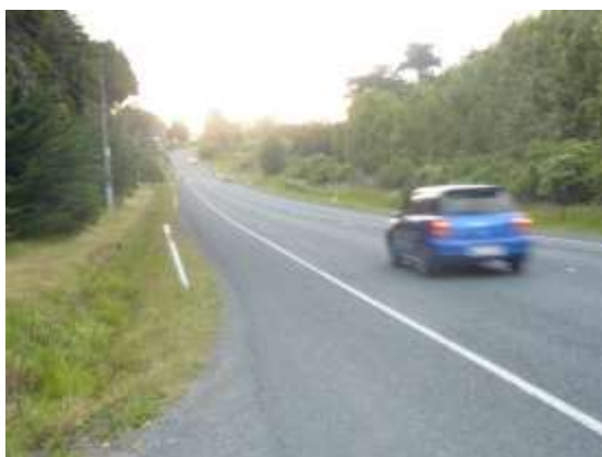
Figure 20: Sealed shoulder, SH16, Akl
