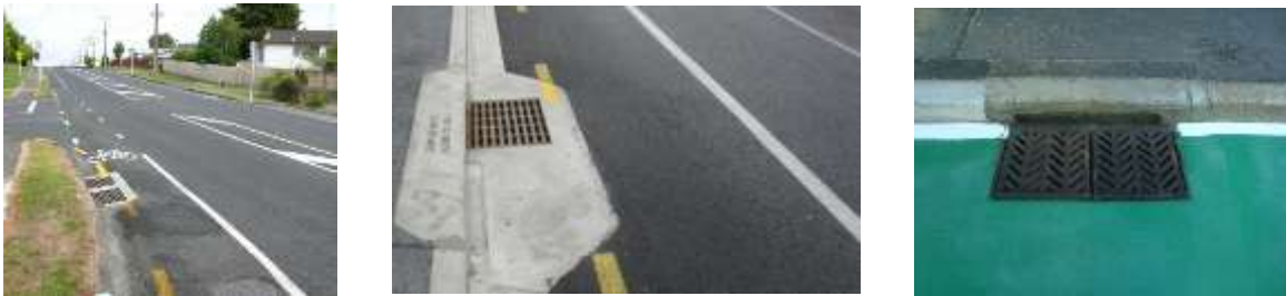
Figure 43: Cycle lane with acceptable grate and lip-less road surface (left to right: Triangle Rd, Ian McKinnon Drive, example from Sydney)
