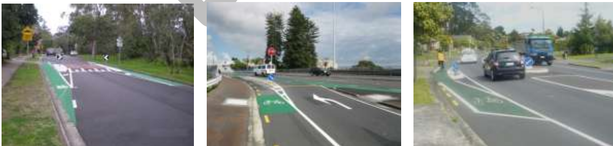
Figure 40: Examples of cycle bypass of speed hump (left, Source: Austroad) and cycle bypass at kerb build outs Ian McKinnon Drive Akl (middle), Summerland Drive Akl (right)
