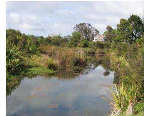
Native wetland plantings on stormwater pond
