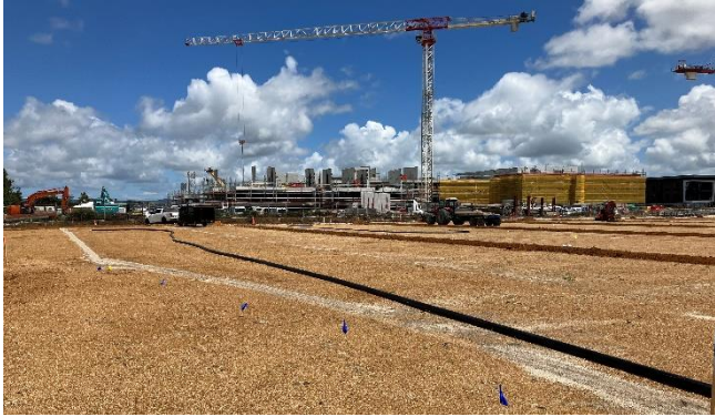
Drainage channels installed in the sportsfields, January 2023.
