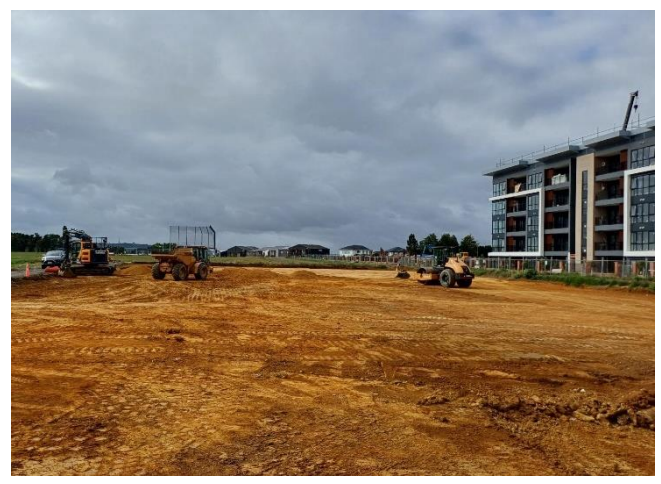
Photo: Earth works for the construction of Fields 4 and 5, March 2024
