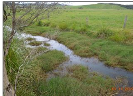
DRAINAGE CHANNEL: POOR FLOW
