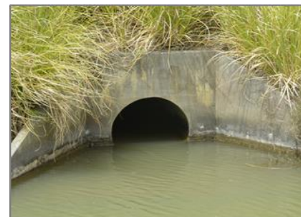
CULVERT: GOOD CONDITION
