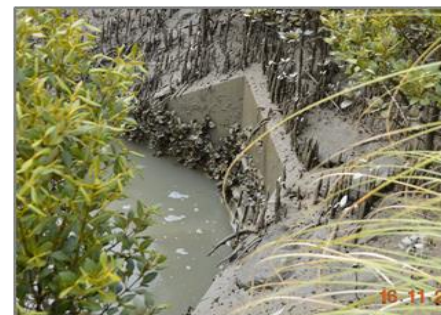
FLOOD GATE: GOOD CONDITION
