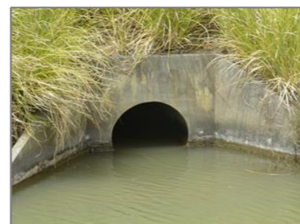
CULVERT: GOOD CONDITION
