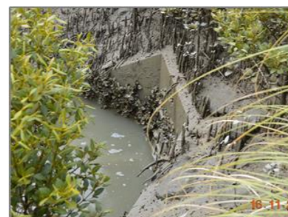
FLOOD GATE: GOOD CONDITION
