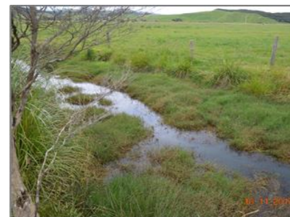
DRAINAGE CHANNEL: POOR FLOW
